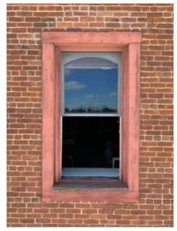
We would like to replace the window, sill and trim with a custom vinyl window from Tri-State Custom Windows. We will wrap the existing sill and trim in metal (and paint it the same color Burnt Red), or if possible, we would prefer to replace the wood trim and sill with Palight (in the same dimensions) also painted in the same color Burnt Red. The exterior color of the vinyl window itself would change to be Beige.
