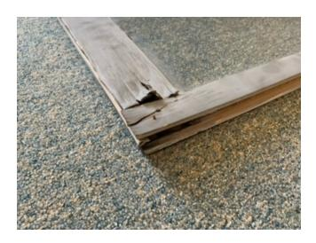
The window sill has significant water damage issues as well.
