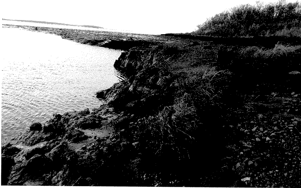
Figure 8: Erosion that occurred in 2015 on west side of harbor
