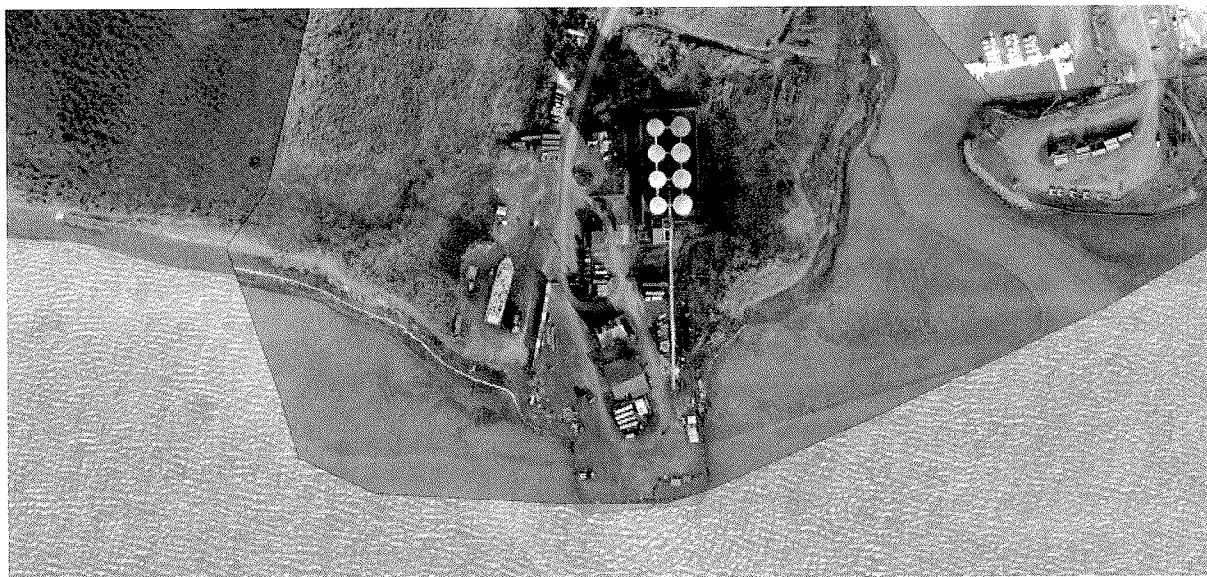
Figure 1: 2016 Aerial Photo of BAF Site
