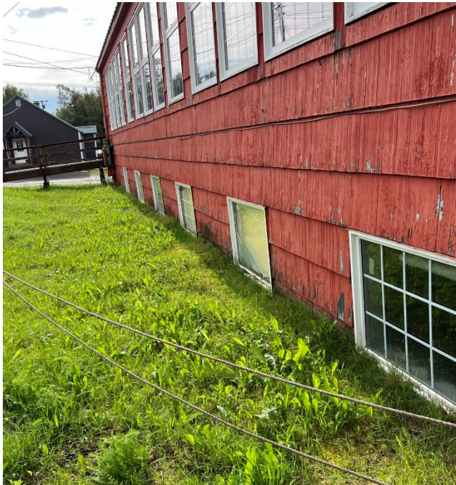
Figure 1: North side retaining wall
