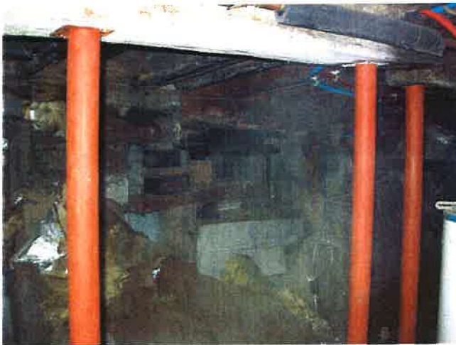
See the stacked up block and timbers for the exterior foundation wall in the distance, note the mold again
