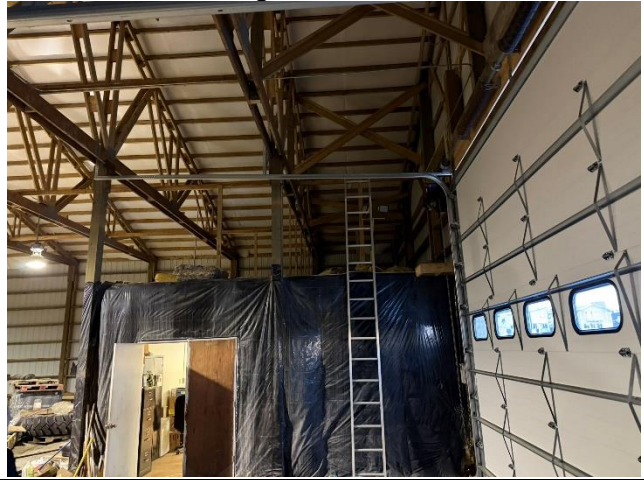
2-Ton Manual Hoist / Insulated Roof
