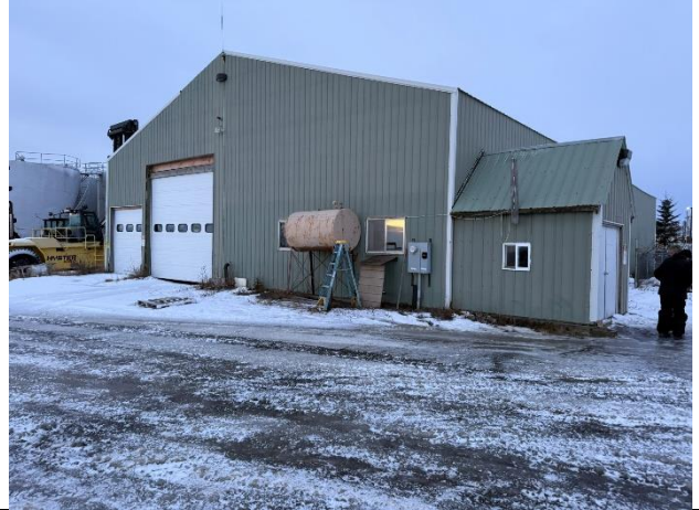
Overhead Door not Flush with Gravel Entry
