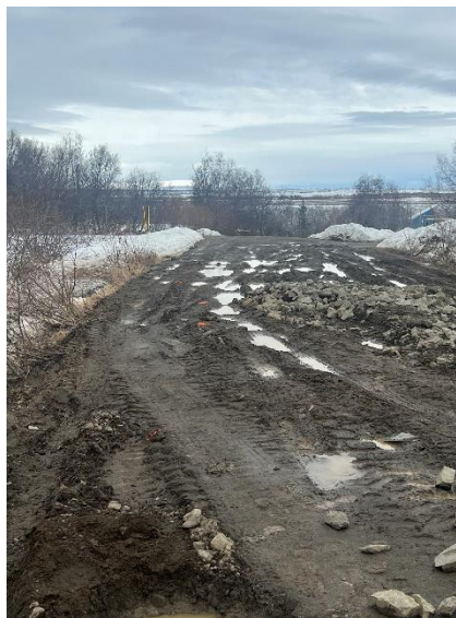
1Road with some shot rock
