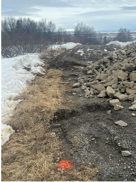
3Road with additional fill
