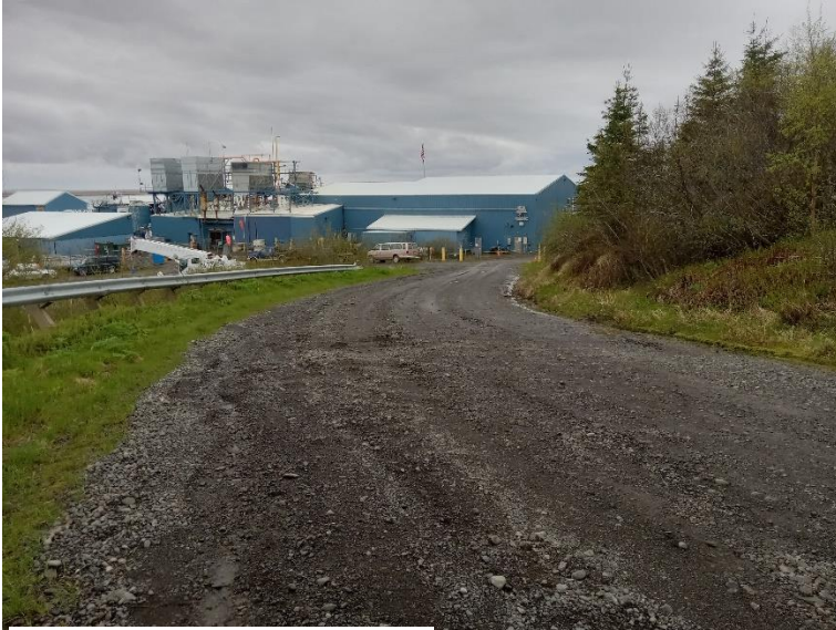
Ditching that needs improvement
