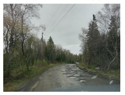
5. Bottom of Sampson Hill, flooding And known culvert failure
