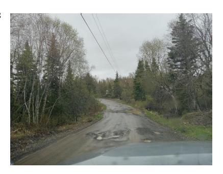
6. Ponding that is an annual issue at the Base of Sampson Hill. Residents living On Squaw Creek Road have filled this Several times with gravel due to Failed culvert and drainage issues Into this low-lying area.
