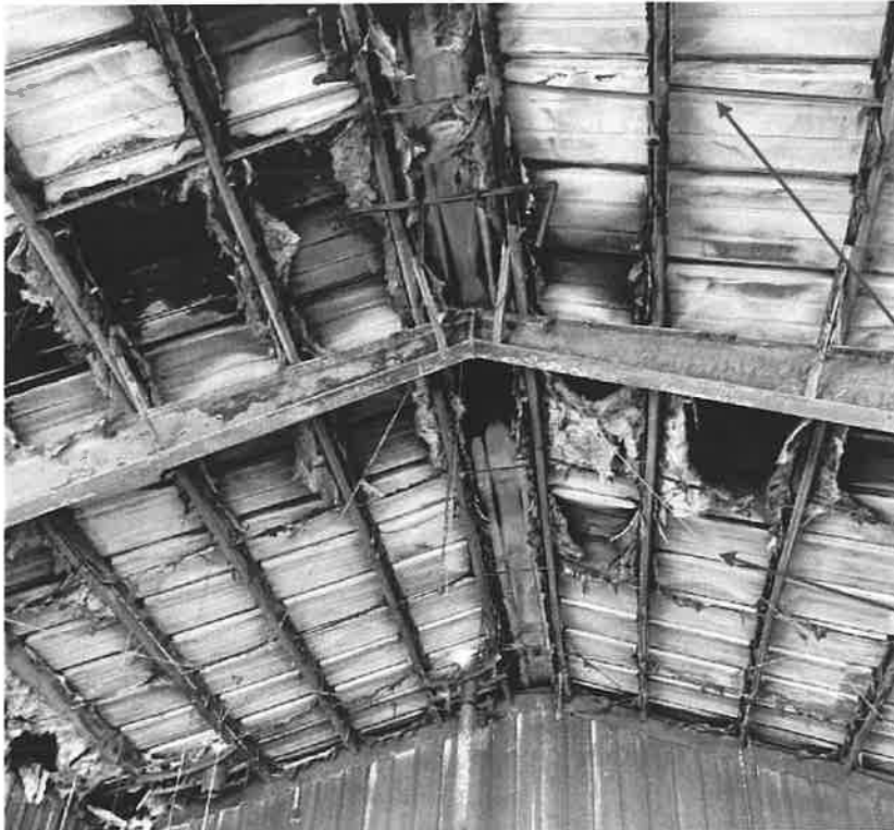
Figure 3: Roof purlins. Bracing indicated
