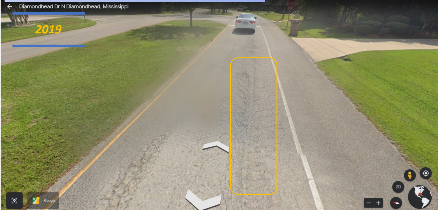
Severe shoving and fatigue cracking at the intersection of Bayou Drive and Diamondhead Drive West in past imagery and present.
