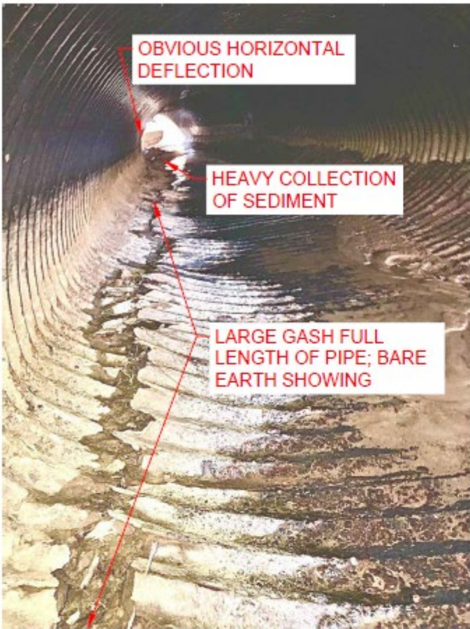
LOOKING UPSTREAM ON DOWNSTREAM CULVERT
