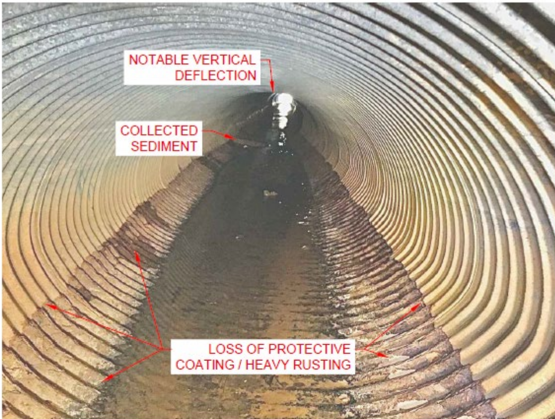
LOOKING UPSTREAM ON UPSTREAM CULVERT
