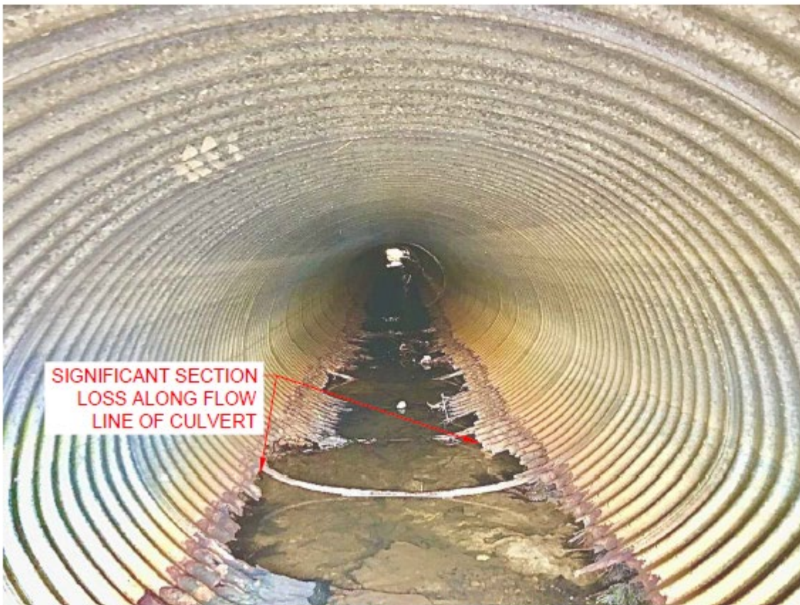
LOOKING DOWNSTREAM ON UPSTREAM CULVERT
