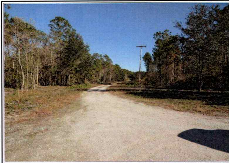
Looking East along Noma Dr (extended) from near the bayou.
