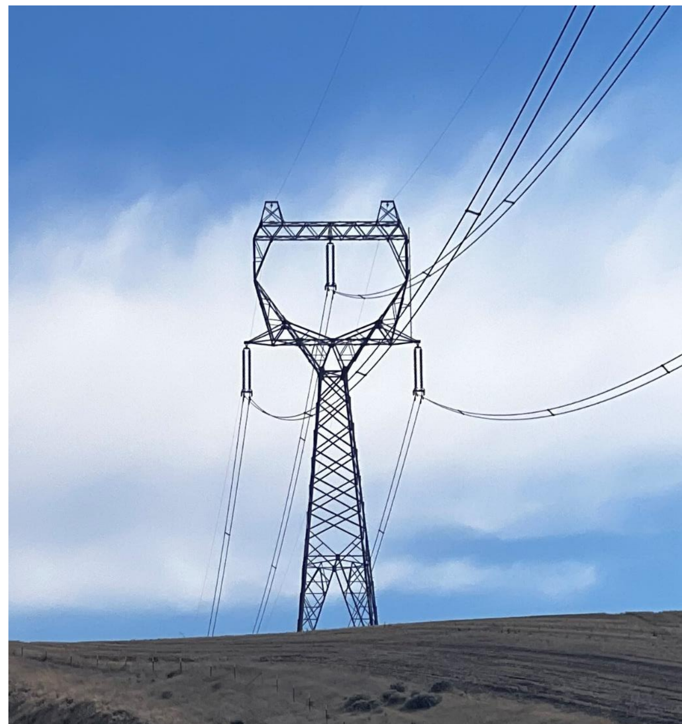
TYPICAL SINGLE CIRCUIT 500-KV TRANSMISSION
