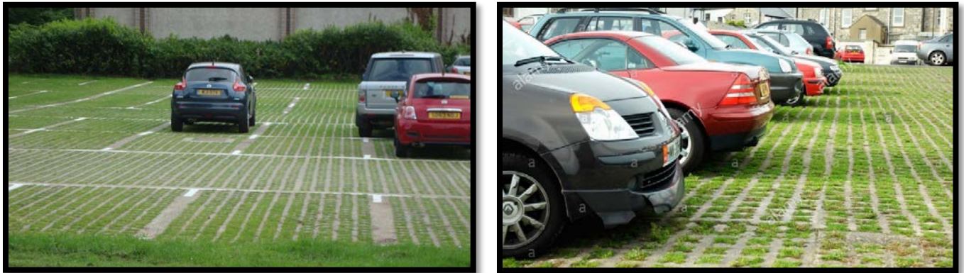
Figure 16 – Applicant's Attachment B - Grass Crete & Sand Crete Paver Examples
