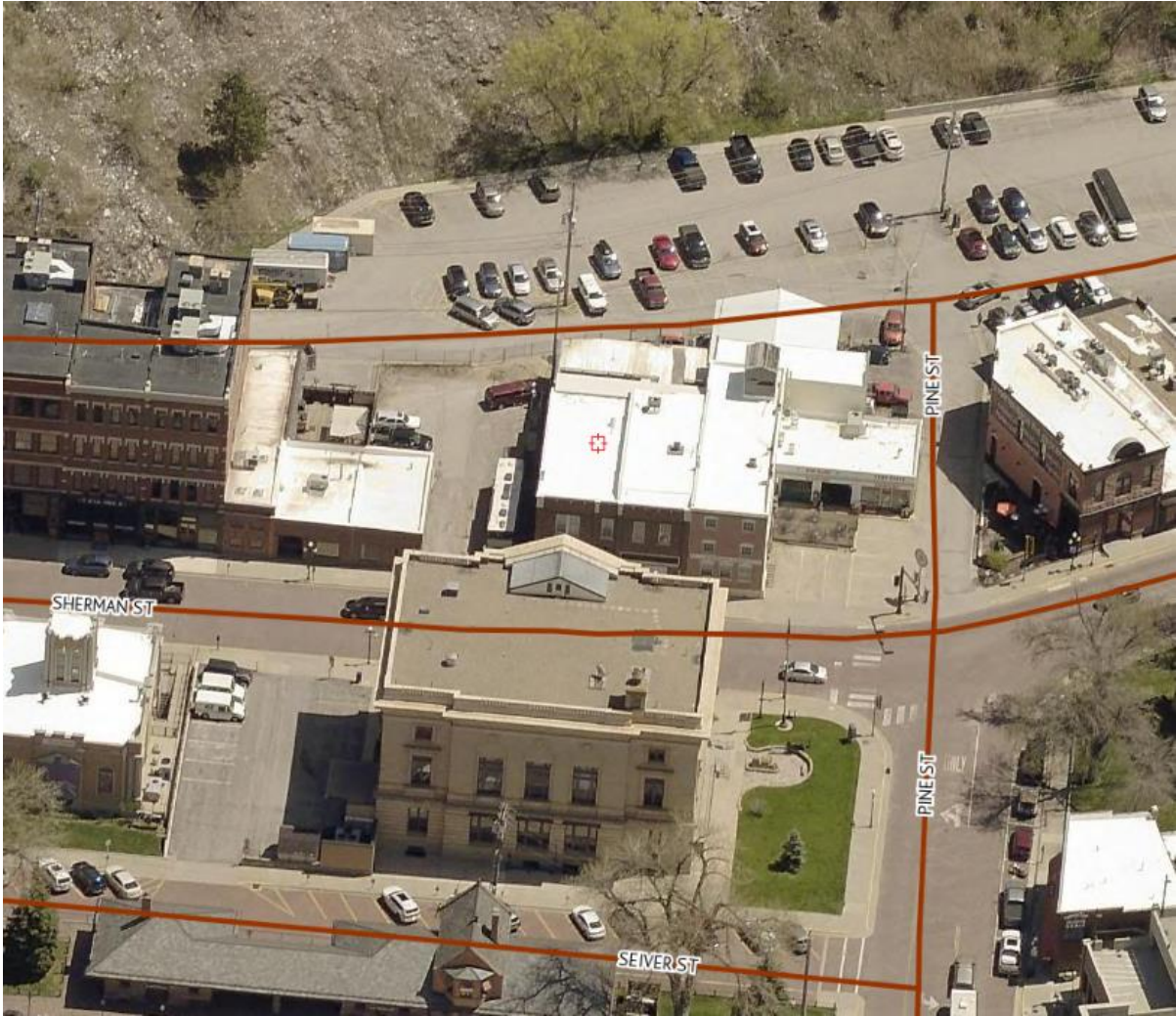
Aerial photo of 65 Sherman Street, Deadwood, SD 57732.
