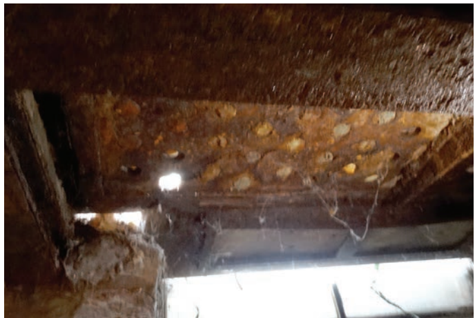
2018: Inside view of sidewalk vault cover. (Winter & Company)
