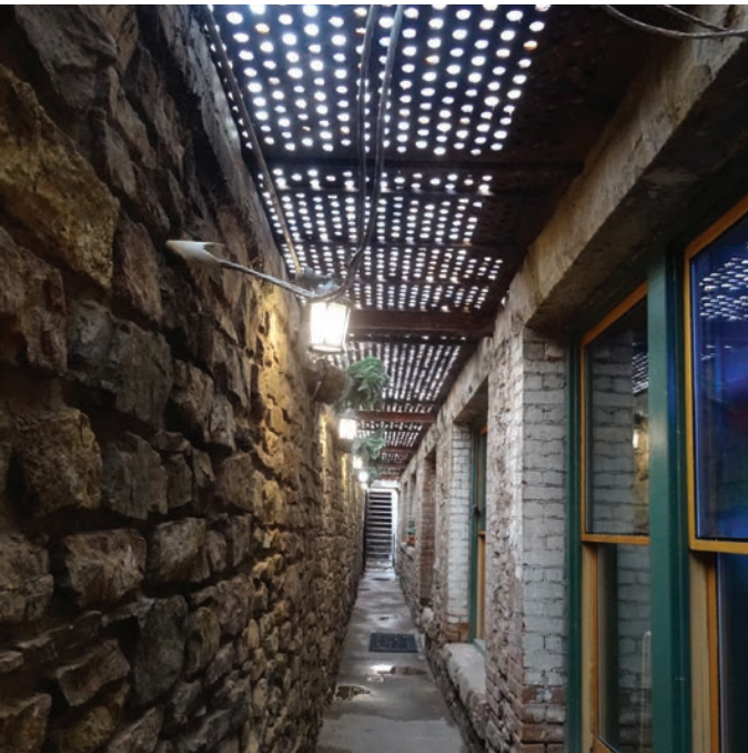
2018: Inside view of restored sidewalk vault cover along Franklin Hotel. (Winter & Company)
