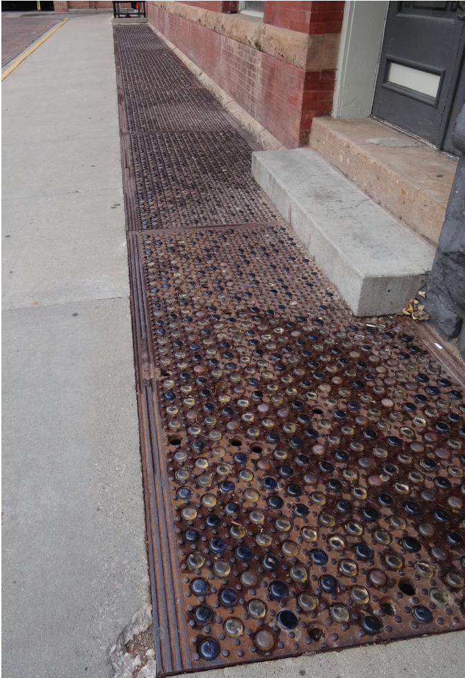
2018: Outside view of sidewalk vault with restored glass pucks. (Winter & Company)
