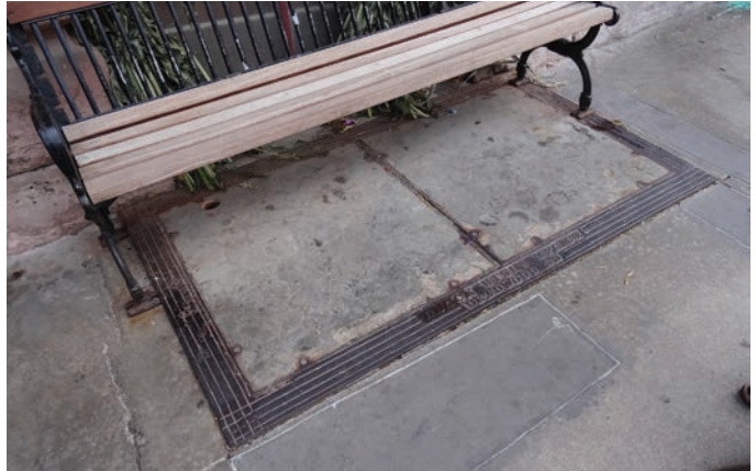
2018: Outside view of sidewalk vault covered with concrete coating. (Winter & Company)
