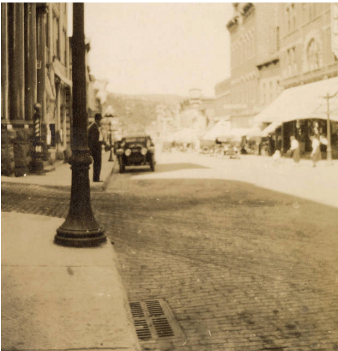
DATE?: Storm sewer grate. Concrete sidewalk with no curb and gutter, brick street. ("2019-10-28-319 storm sewer grate SDDA.jpg")
