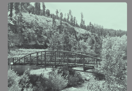
Bridge Over Whitewood Creek
