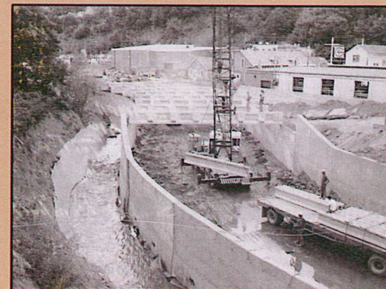
Below: September 11, 1967 box culvert installation.
