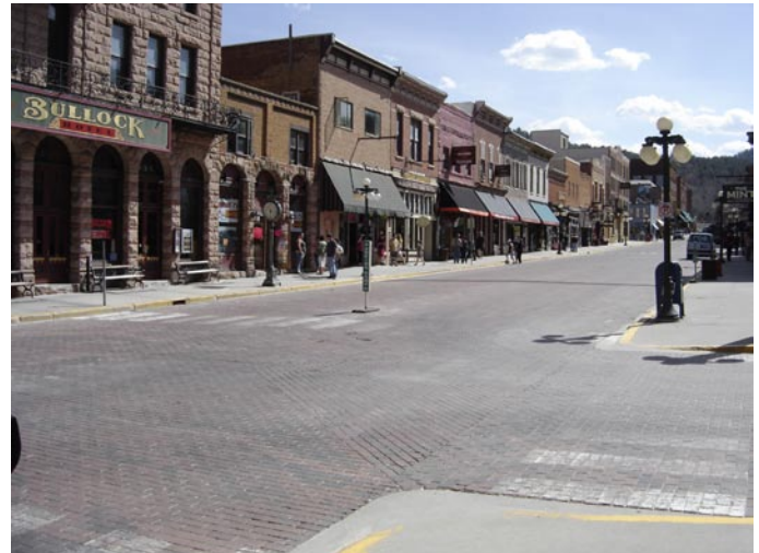
Sandy soils and the underlying brick pavers give pavement markings a short life. Markings were reapplied during the Summer of 2008.
