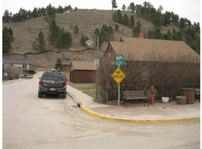
The lack of curb ramps makes an otherwise adequate sidewalk inaccessible for some users. The plan calls for the construction of 46 new curb ramps including here at the intersection of Cliff Street and Burlington Street.
