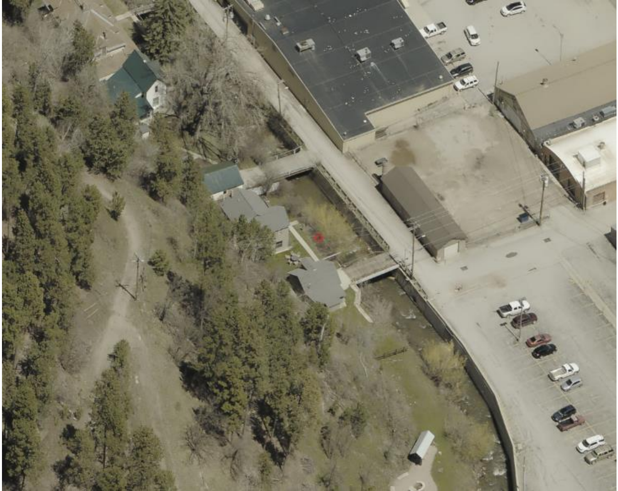
Aerial view of 36 Water Street.
