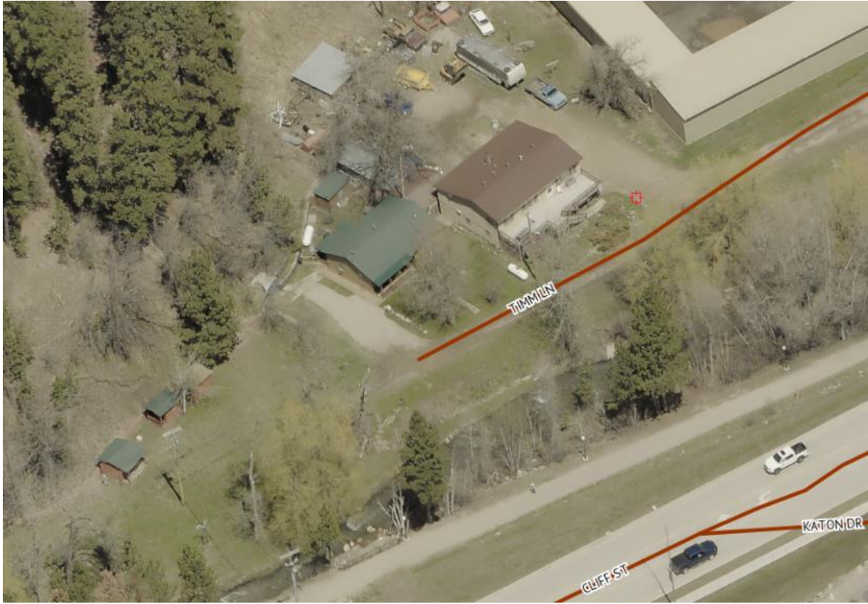
Aerial view of 140 Timm Lane, Deadwood, SD 57732.
