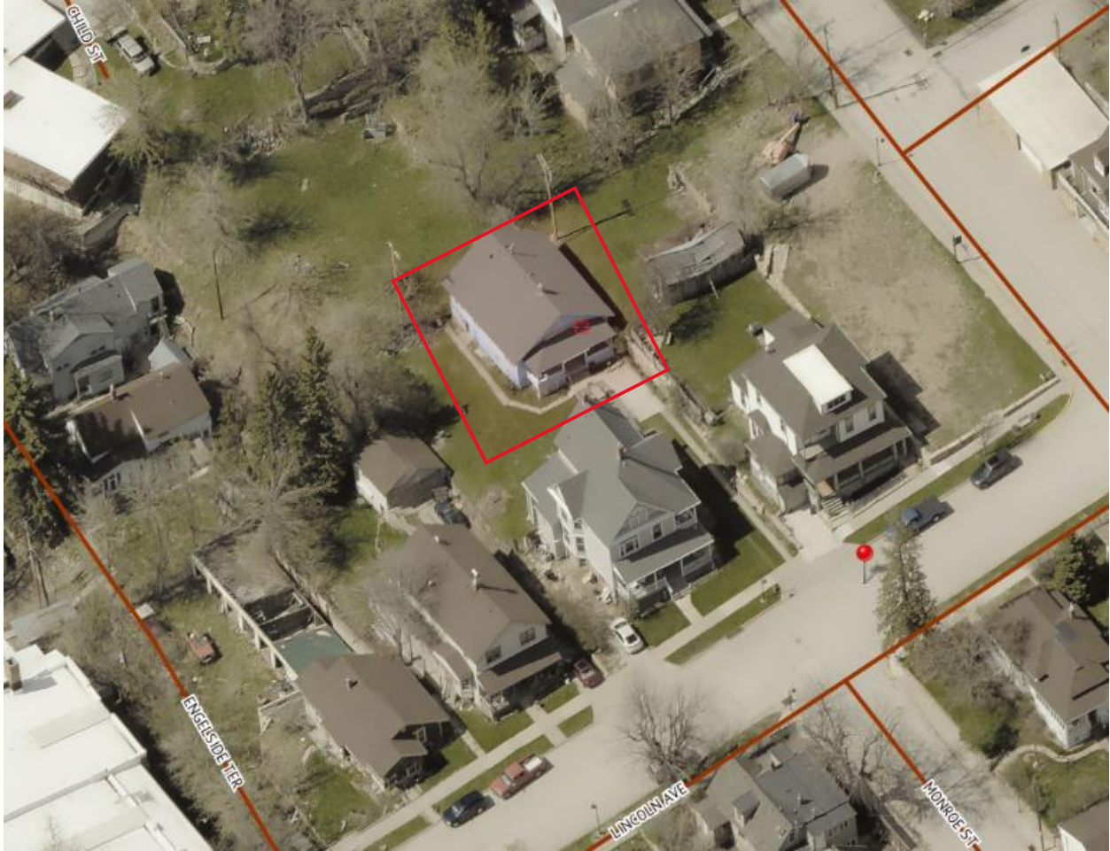
Aerial view of 25 Lincoln Ave, Deadwood, SD 57732.
