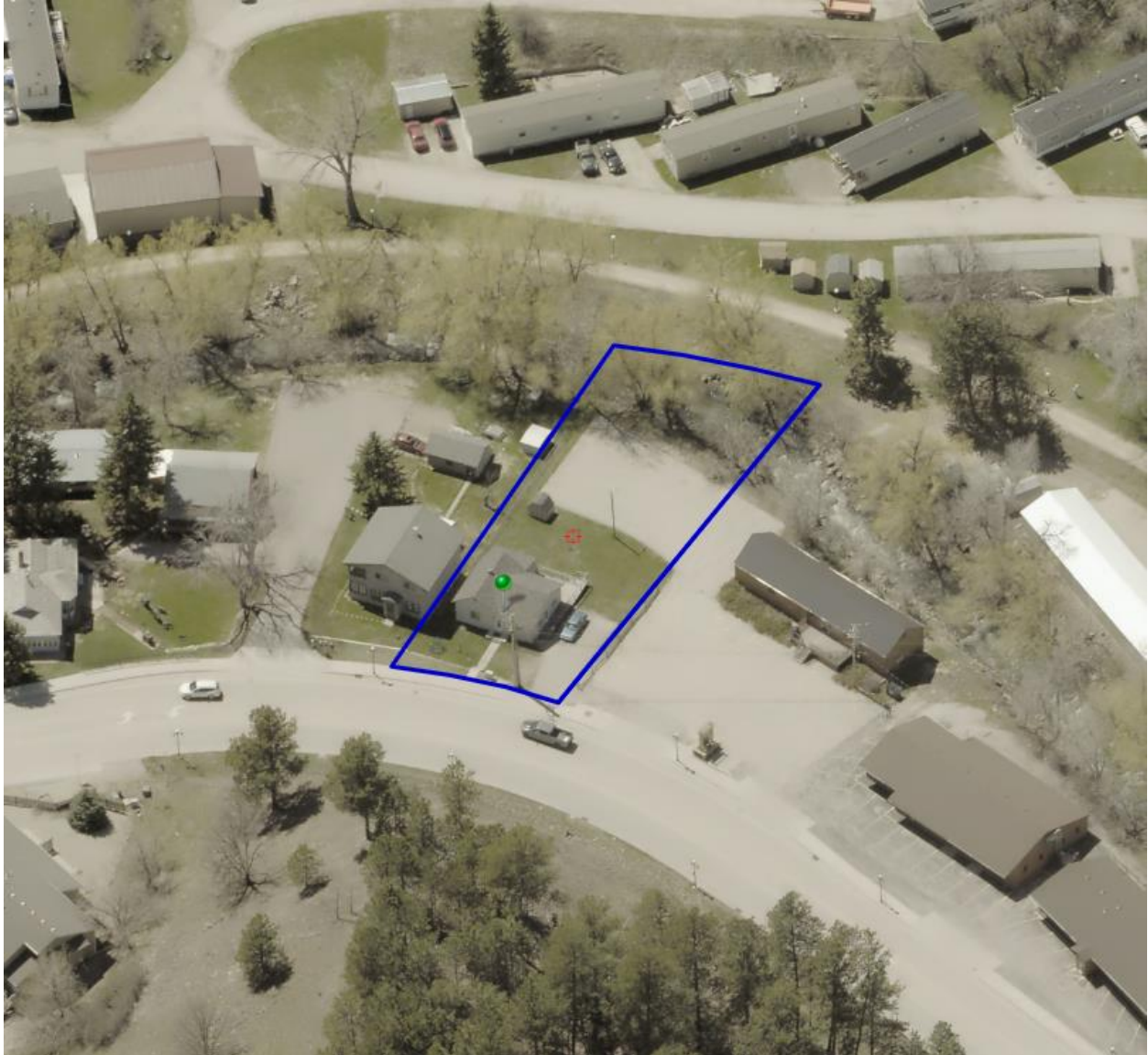
Aerial view of 64 Cliff Street, Deadwood, SD 57732.
