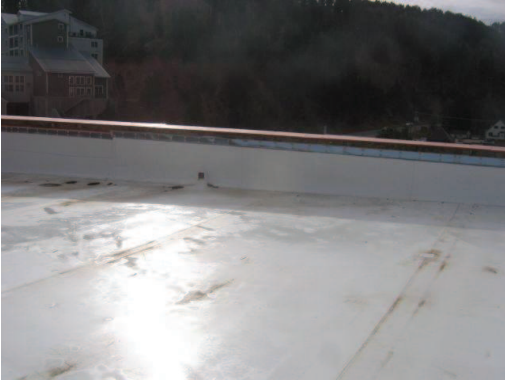
Photo No. 37: South parapet wall.
