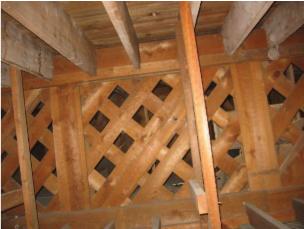
Photo No. 28: Interior panel of subject girder truss.
