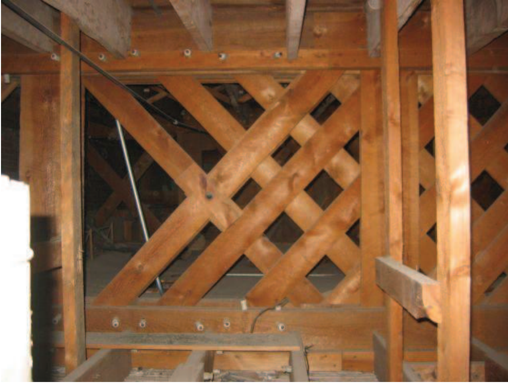
Photo No. 29: View of girder panel at south end of girder truss.
