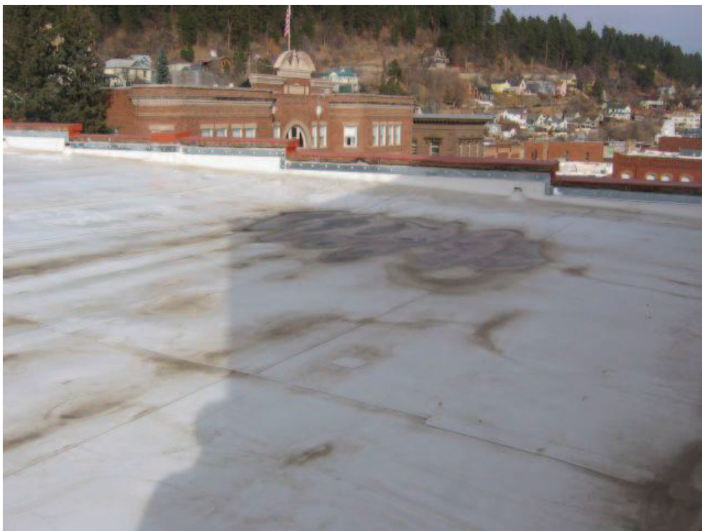
Photo No. 34: North parapet wall at girder truss.
