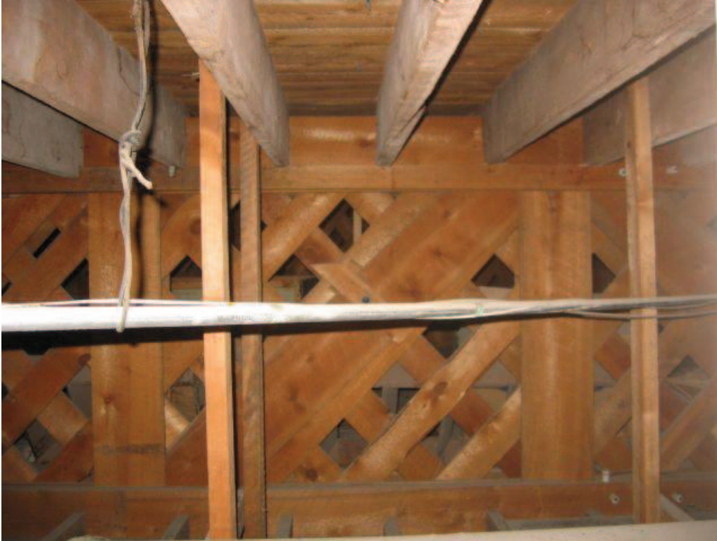
Photo No. 27: Interior panel of subject girder truss.
