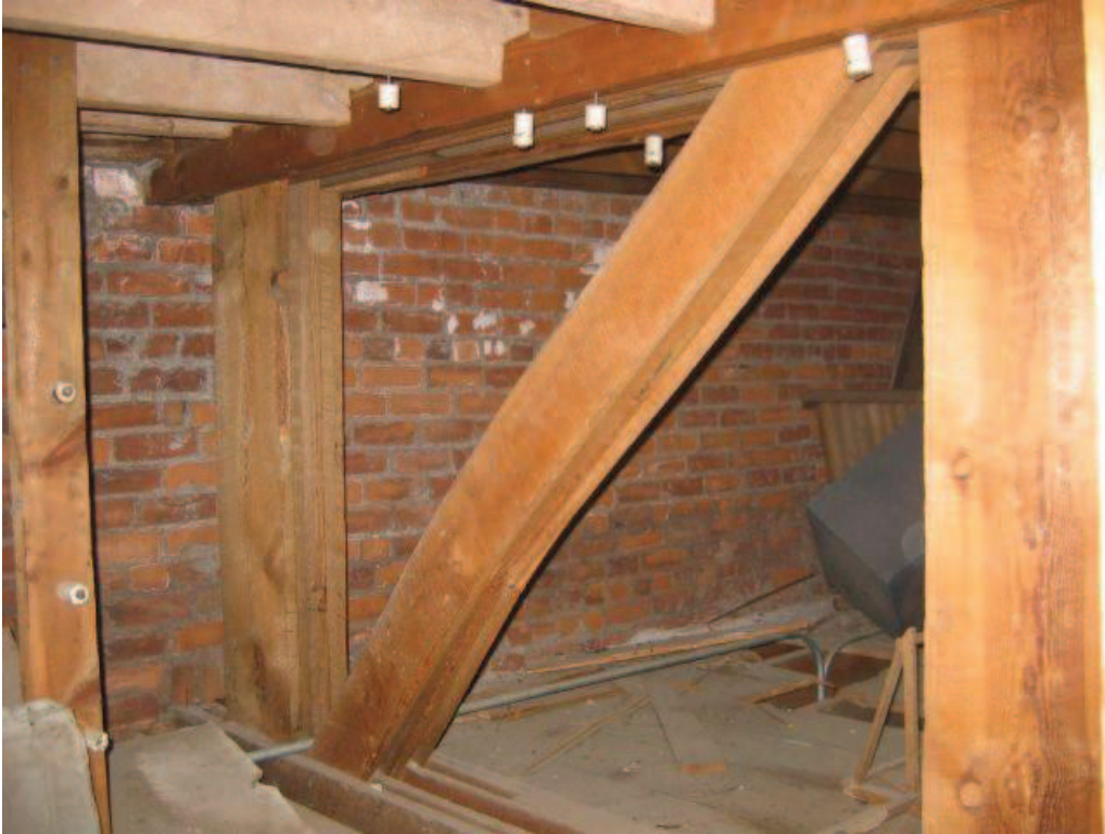
Photo No. 15: Breakage of the diagonal at south end of girder truss.
