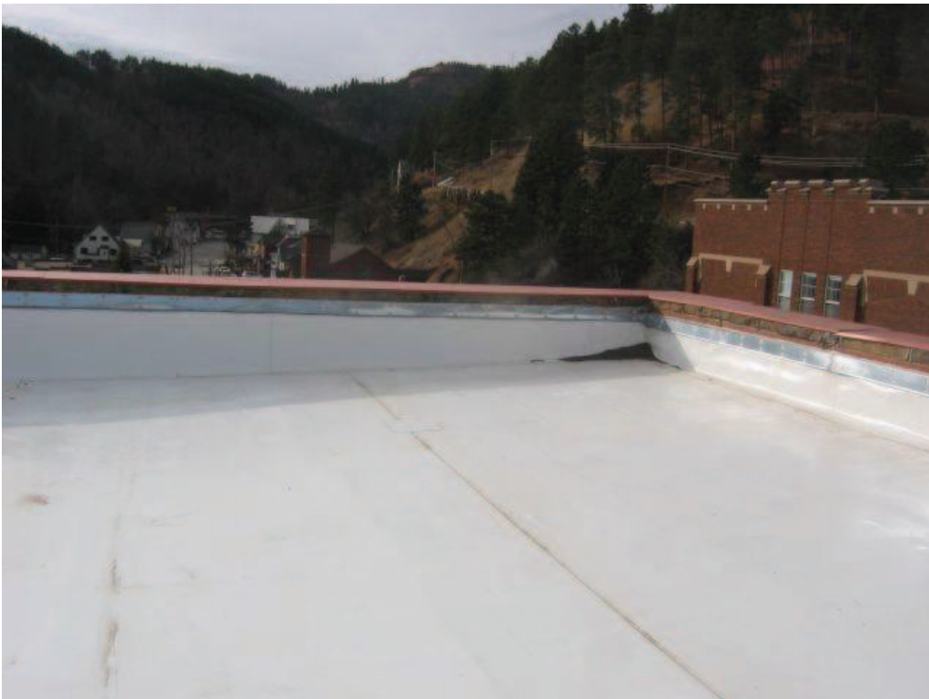
Photo No. 38: Southwest corner of roof and parapet.
