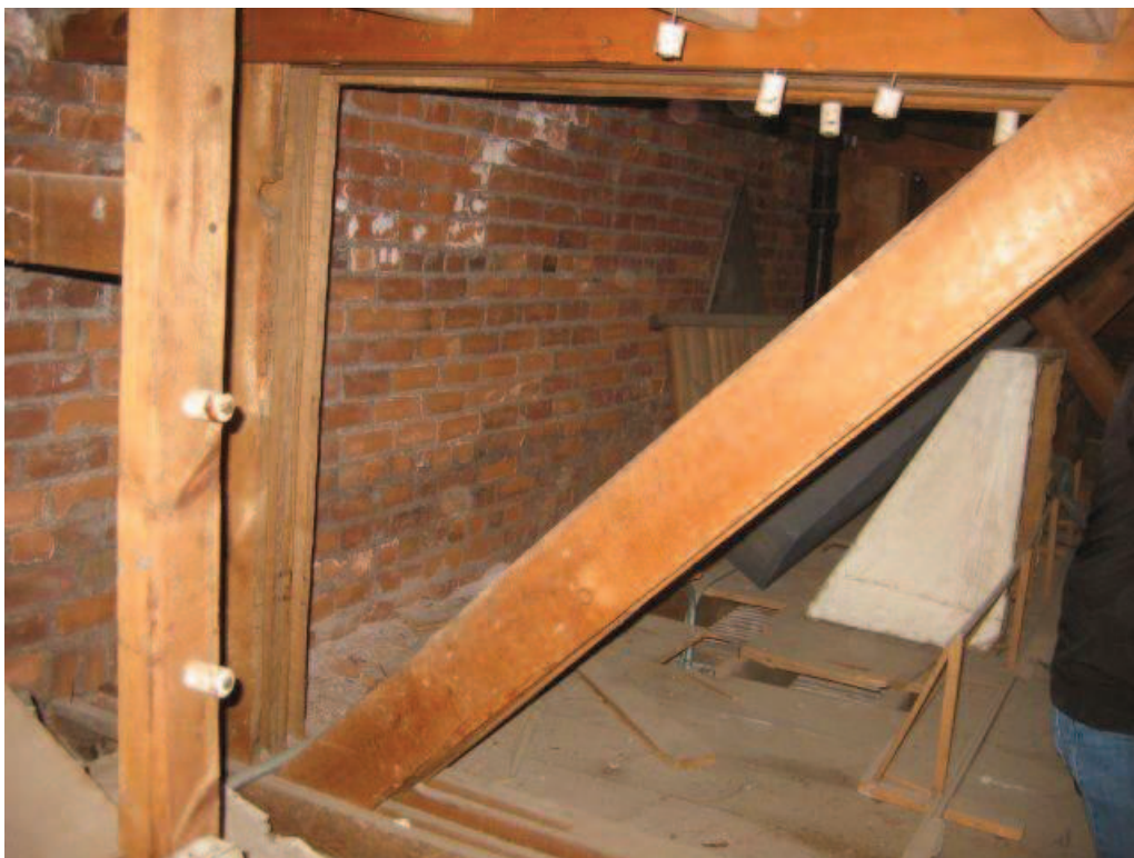
Photo No. 14: Diagonal chord member at south end of girder truss.
