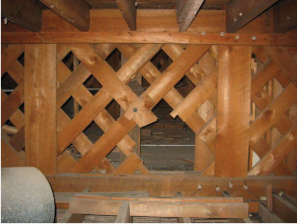
Photo No. 25: Interior panel of subject girder truss.
