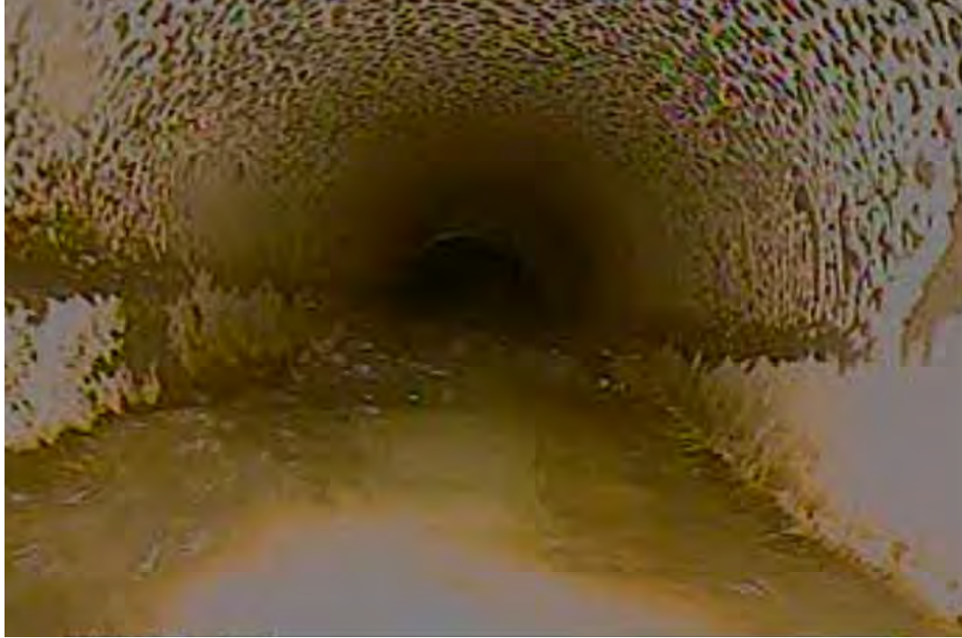
Picture 3 Example of sag in sewer main
