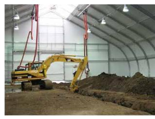
A temporary enclosure system is one method to extend construction activity into winter season.
