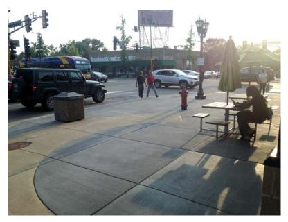
Figure 4. Colored concrete is used to highlight this bumpout, which incorporates ADA ramps, a street light, fire hydrant, trash can and plenty of seating. It is important to note that while this bumpout incorporates similar ideas to those proposed for Deadwood, the colored concrete is used in a much different way than might be considered for Deadwood's Main Street.
