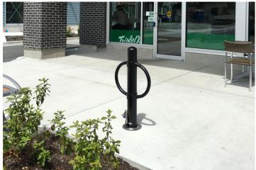
The bike locking arms can be used to lift a bollard installed with a removable mounting.
