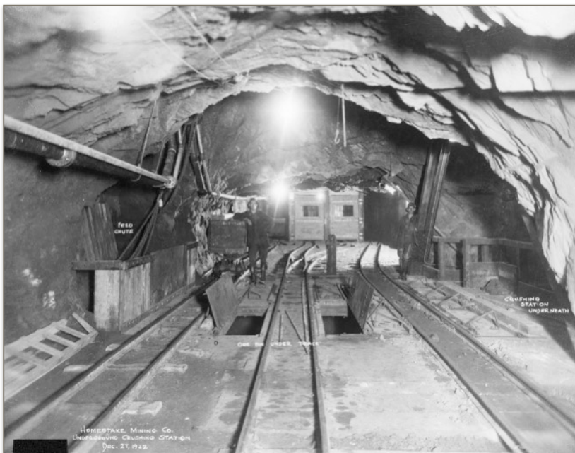
Underground crushing station, 1922.
