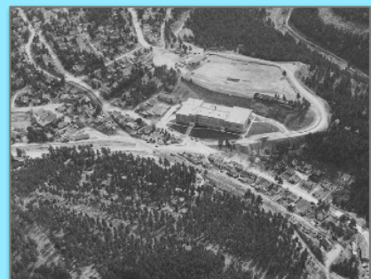
Aerial view of Lead High School in 1943
