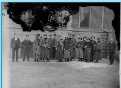
Damaged glass plate of unknown group
