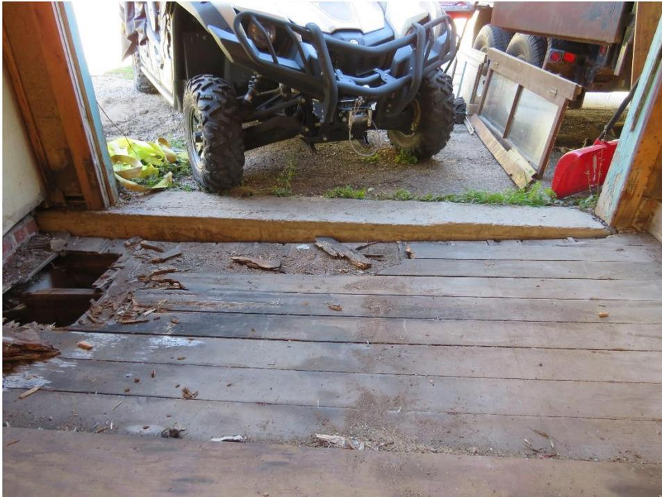
Photograph showing how the garage floor has sank, and is unlevel due to the deterioration. The decking in this section actually moves when you walk on it.
