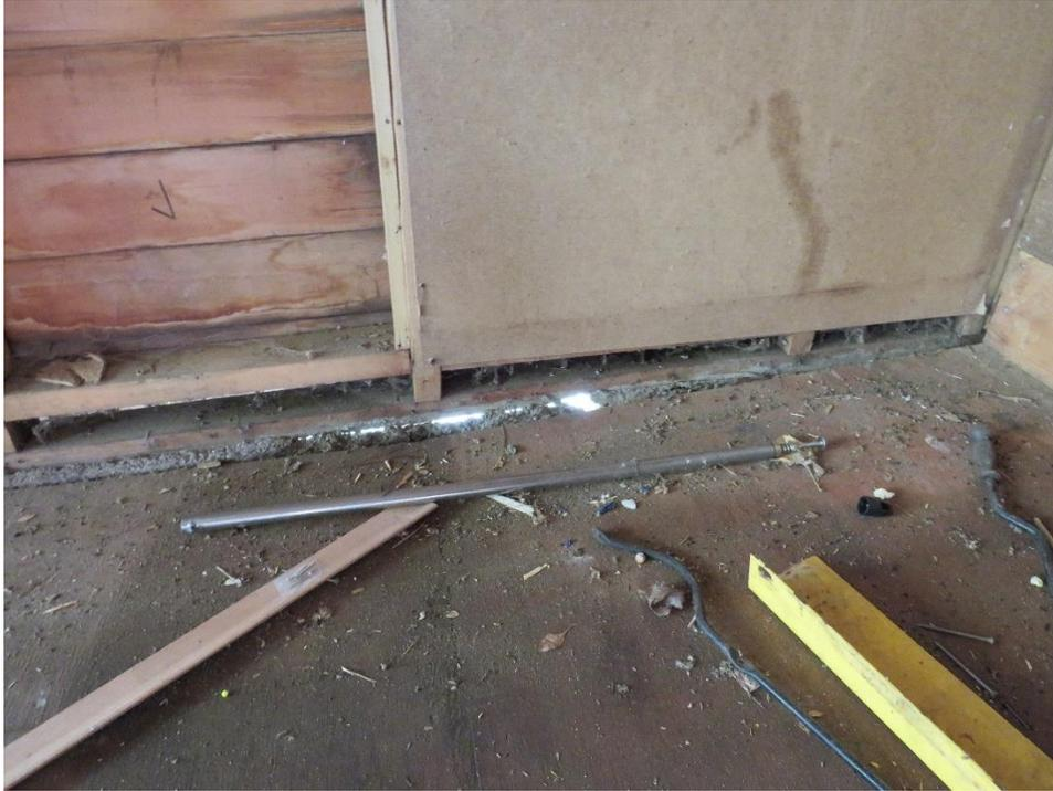
This photograph shows where the structure is off the foundation as you can see light through it.
