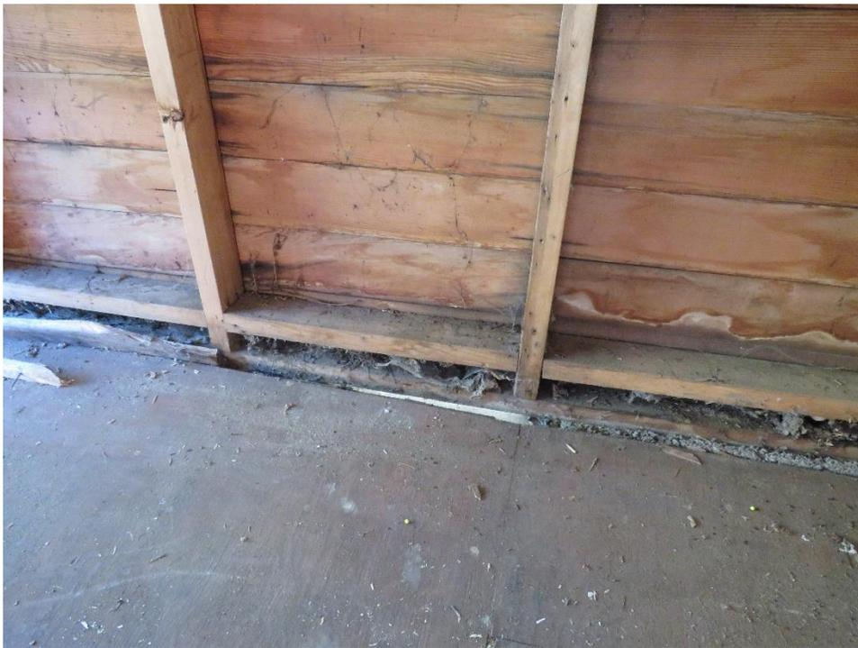
This photograph shows the foundation pulled away from floor and light showing through.
