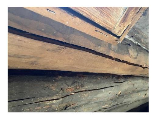
These three photos are the logs needing replaced under the loft window. Plans are to install a double hung window
