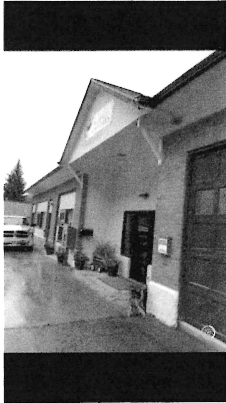
Front of building Current
