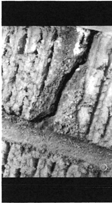
Brick Restoration of brick. Masonry caulked (GREY)
