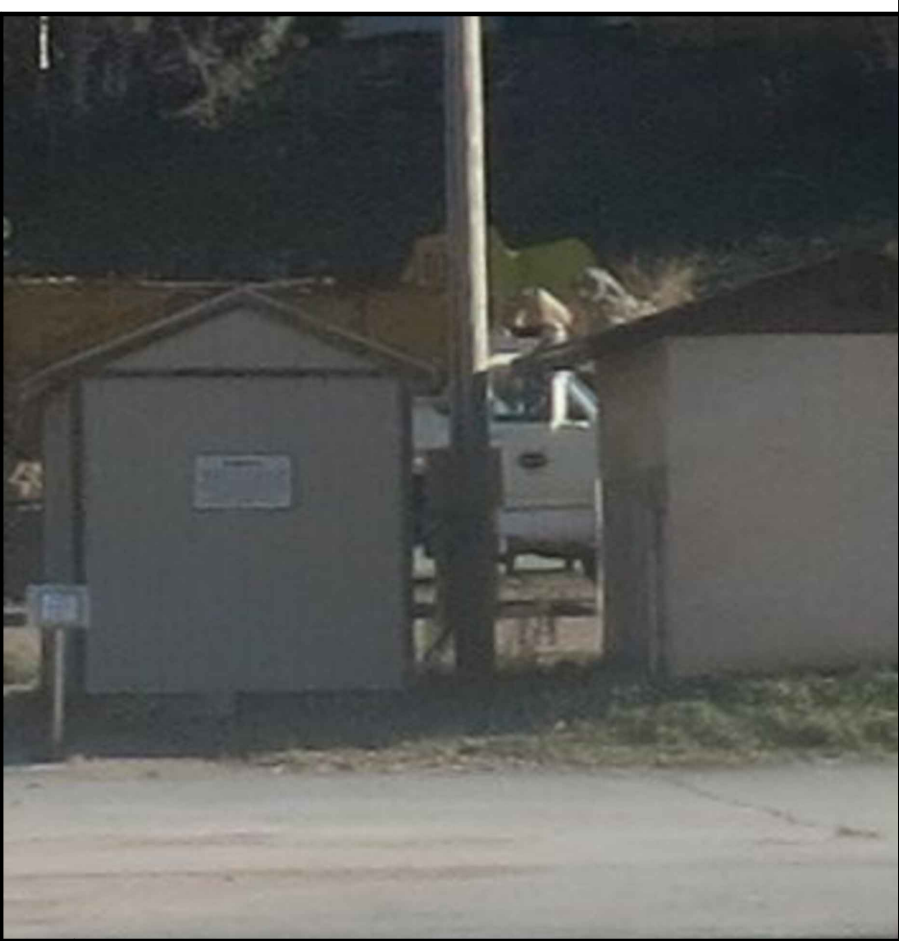
D OVERVIEW OF SITE
