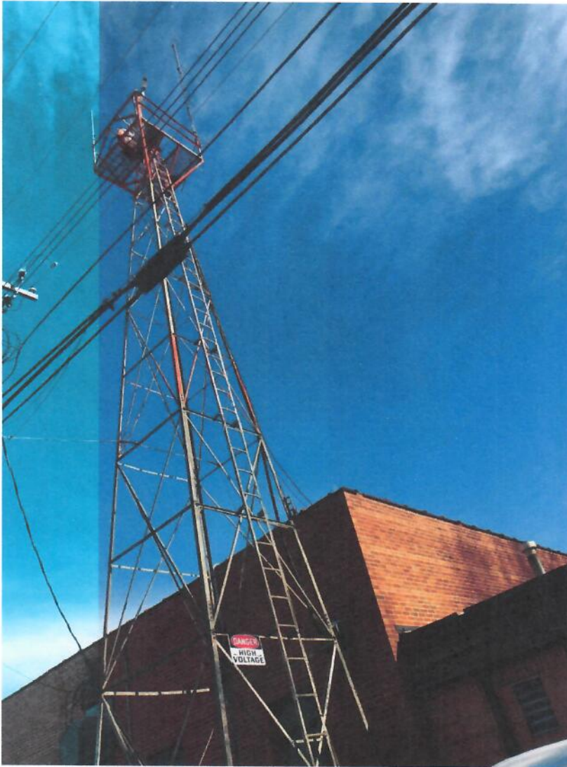
Source: Staff Photo, West Façade (center alley view), January 26, 2026.
