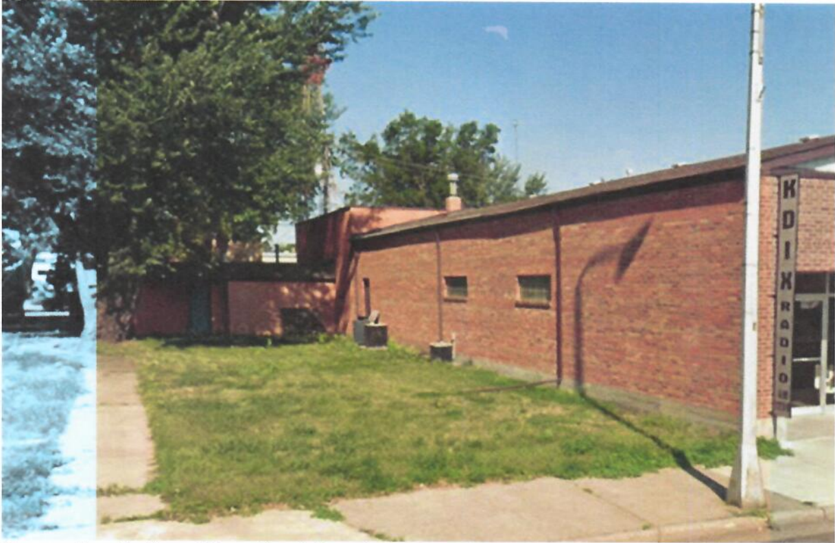
Source: Google Street View, South Façade, August 2019
