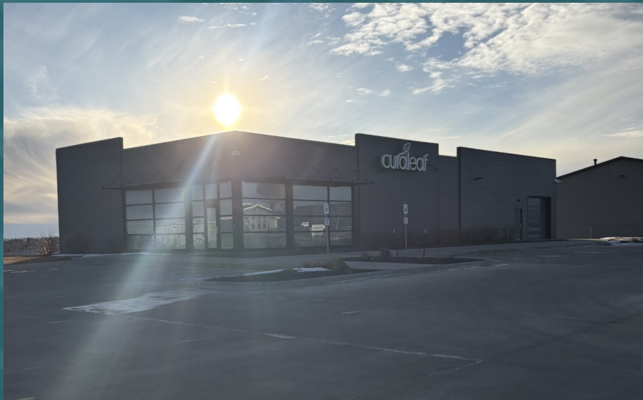
Front of building (view from Northeast)
