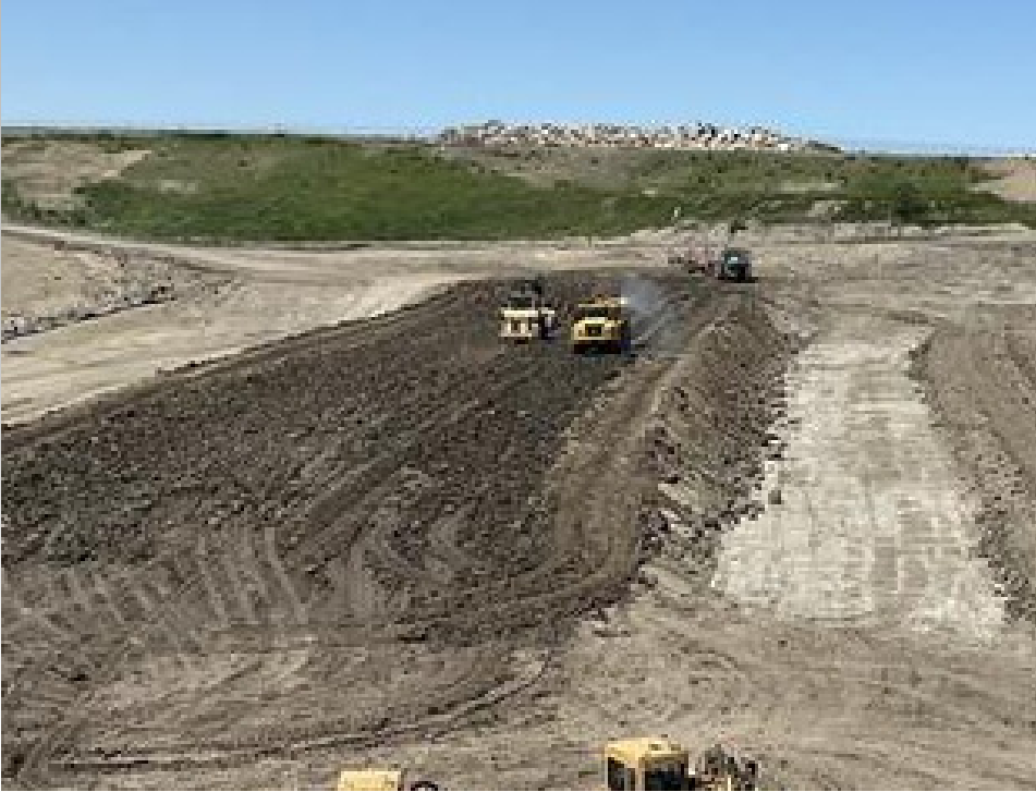
Above: Water truck spraying water on site
