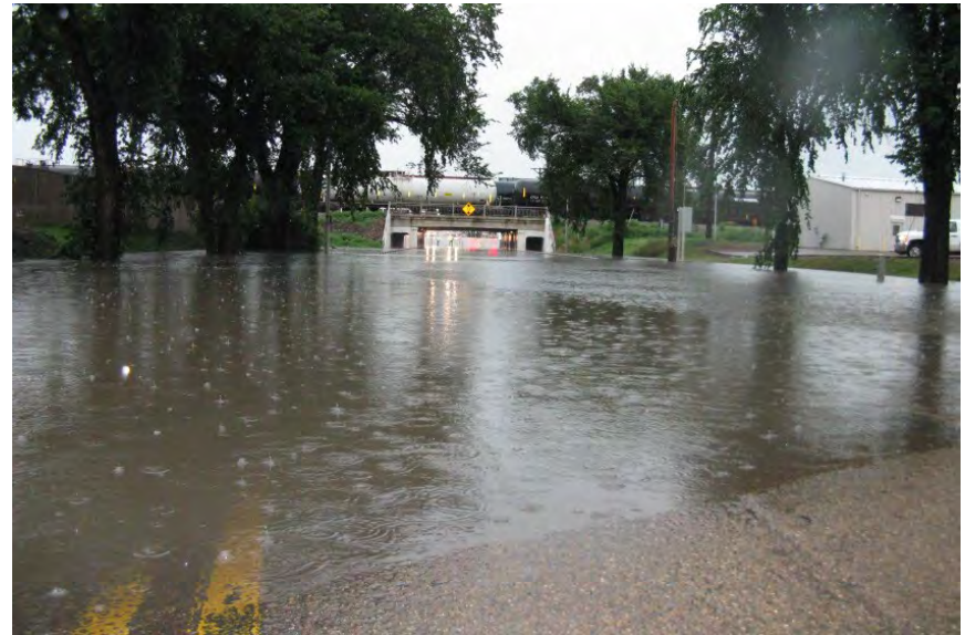
The 3 rd Avenue underpass in Dickinson flooded during heavy rains in 2011. The City is working to make municipal infrastructure more resilient. Image Credit: The Dickinson Press
