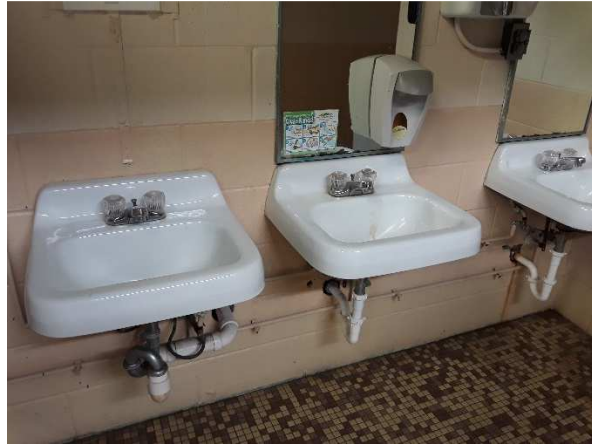
Lavatories – Pool Locker Room
