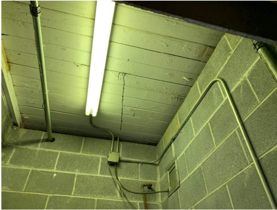
Photograph J: Building A Termite Infestation
