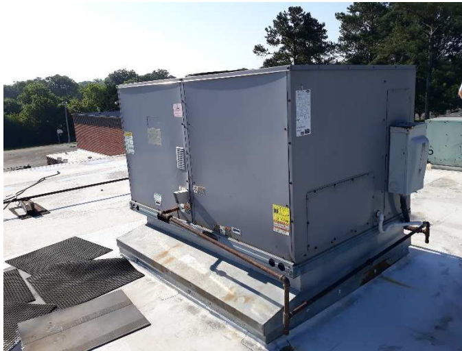
Replacement Multipurpose Rooftop Unit
