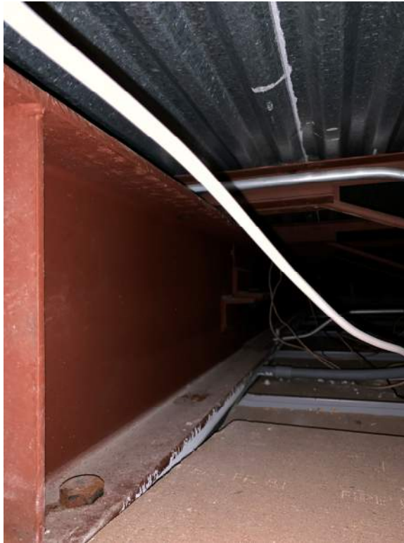
Photograph S: Building C Floor Framing
