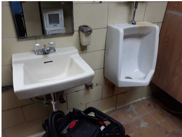
Typical Toilets – Original Building
