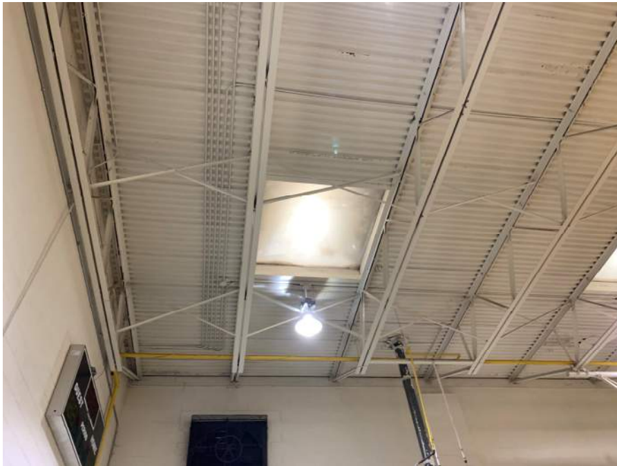
Photograph K: Building B Roof Framing Over Gym Area (Looking North)
