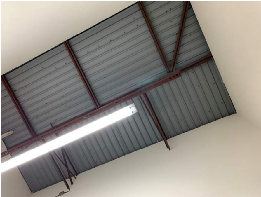
Photograph T: Building C Roof Framing
