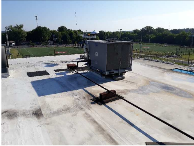
Condensing Unit for Administration Area
