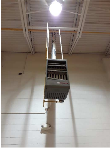
Typical Unit Heater for Gym
