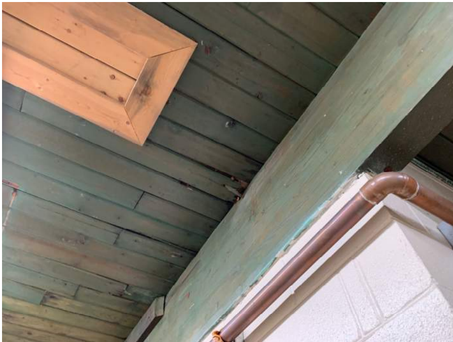
Photograph B: Building A Roof Framing Over Pool Area (Looking North)
