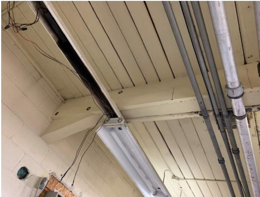
Photograph M: Building B Roof Framing Over Storage Room #2 (Looking North)
