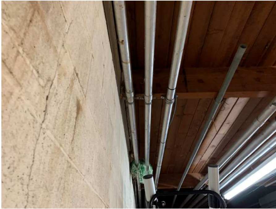
Photograph L: Building B Roof Framing Over Storage Room #1 (Looking East)
