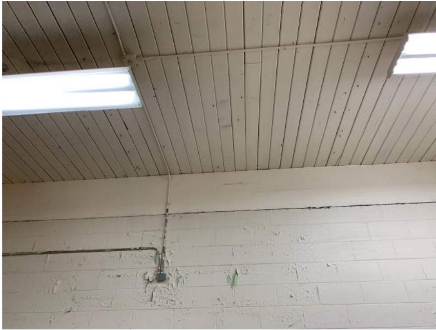
Photograph A: Building A (South End) Roof Framing (Looking South)
