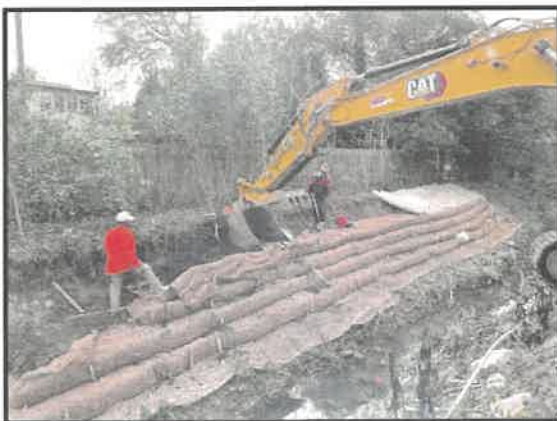
Concept: Bio-D Block Installation
