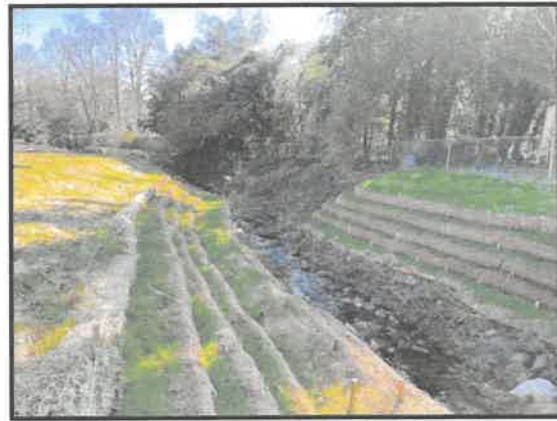
Concept: Bio-D Block Final Condition
