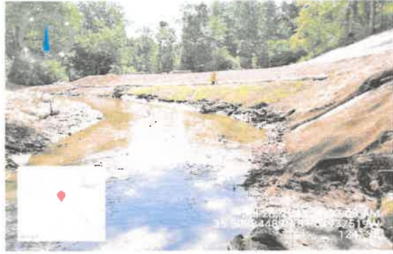
Re-routed and stabilized with in-stream structures
