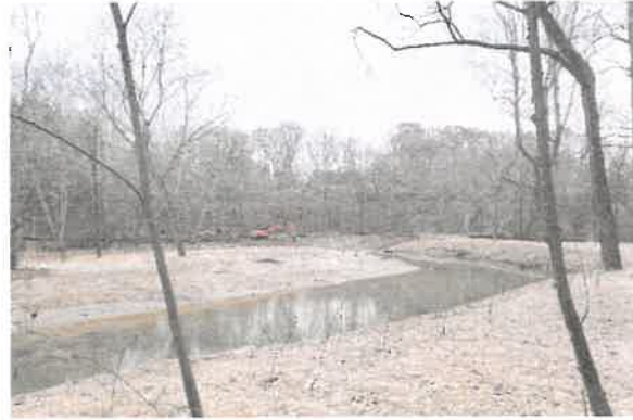
Re-routed stream away from gas line
