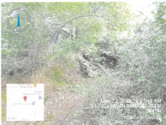
Existing Condition: Looking Upstream
