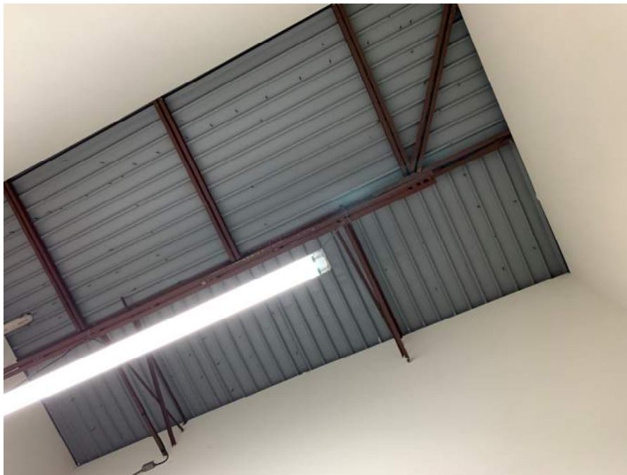
Photograph T: Building C Roof Framing
