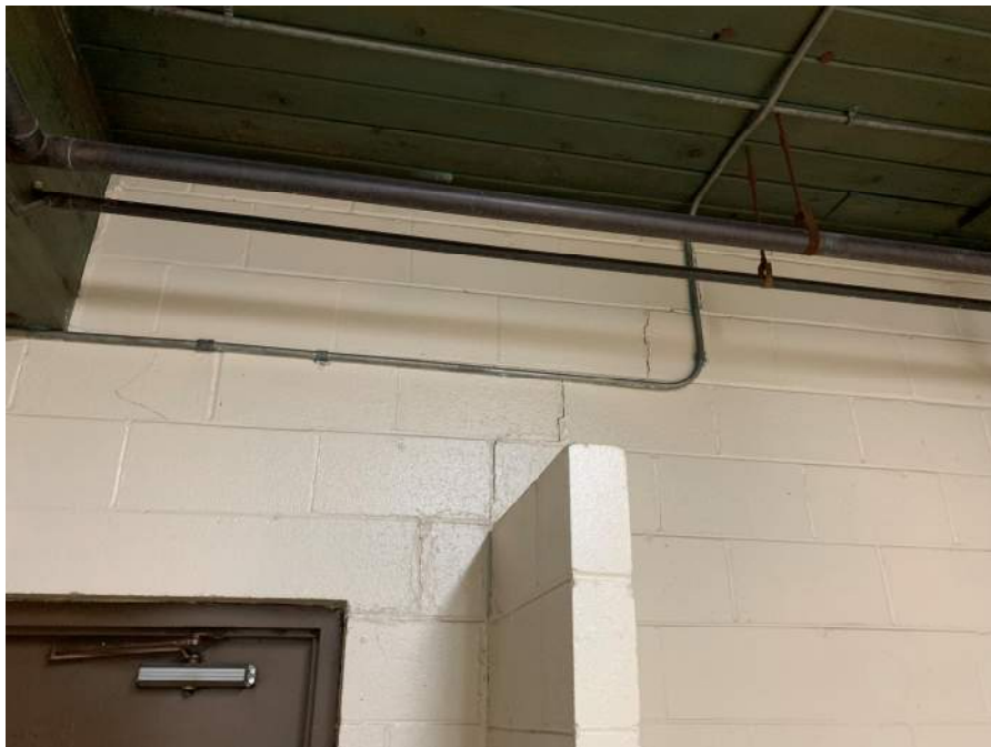
Photograph D: Cracks on Building A Men's Restroom CMU Wall #2
