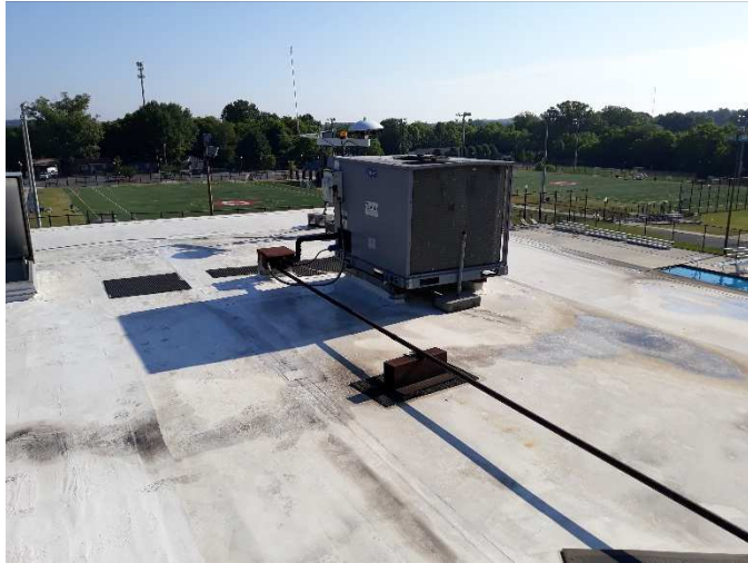
Condensing Unit for Administration Area
