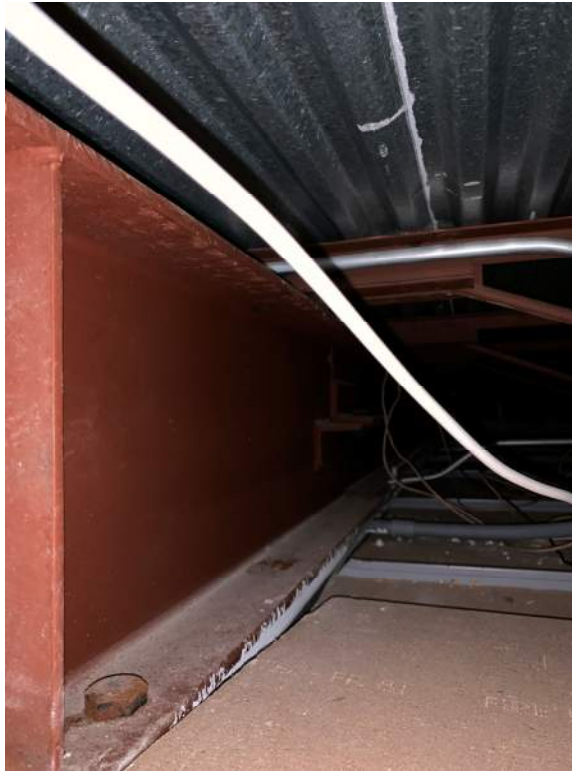
Photograph S: Building C Floor Framing
