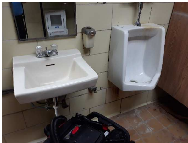
Typical Toilets – Original Building
