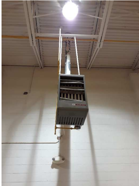
Typical Unit Heater for Gym
