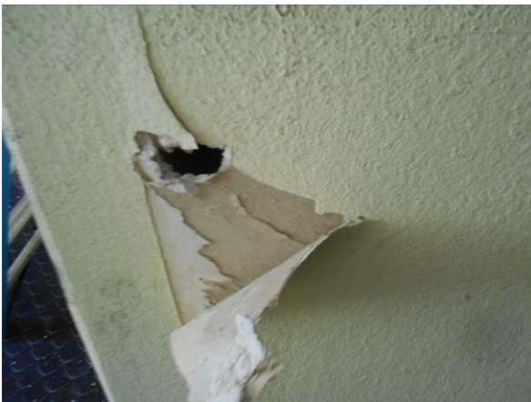
Photo #17 View of the ACM joint compound (HA-27) and textured wall surface in guest rooms.
