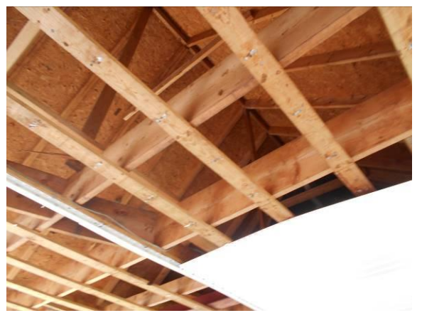
Photo #22 View of wood roof rafters and decking.
