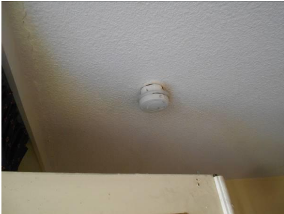
Photo #19 View of the ACM spray applied acoustical texture (HA-33) on ceiling in guest rooms
