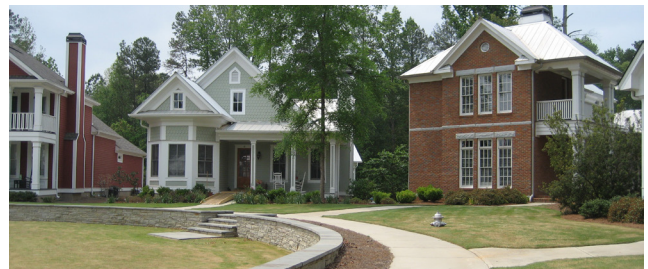
Figure 25 Source: Hall Consulting, Inc.
