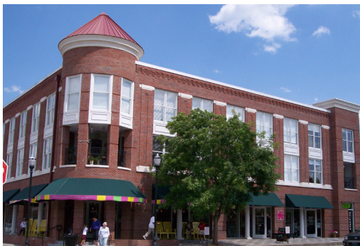
Figure 38 Source: Hall Consulting, Inc.
