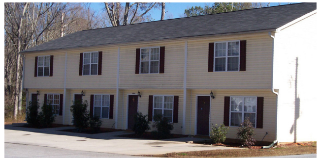
Figure 26 Source: Hall Consulting, Inc.
