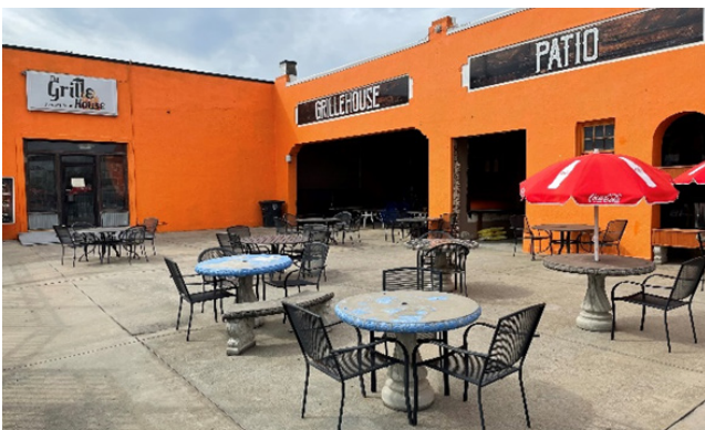
Figure 30 Source: Hall Consulting, Inc.
