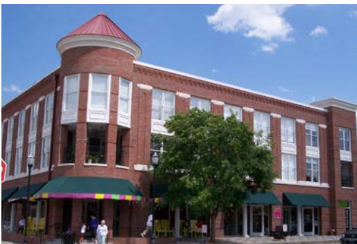
Figure 38 Source: Hall Consulting, Inc.
