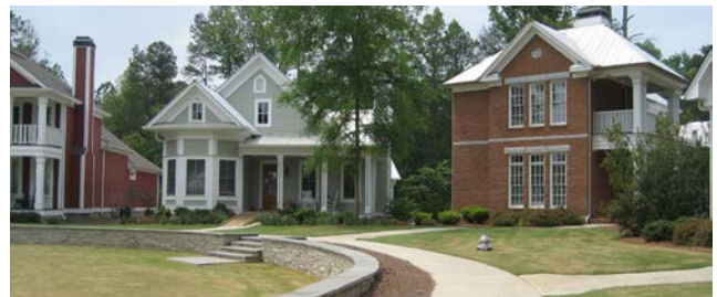
Figure 25 Source: Hall Consulting, Inc.
