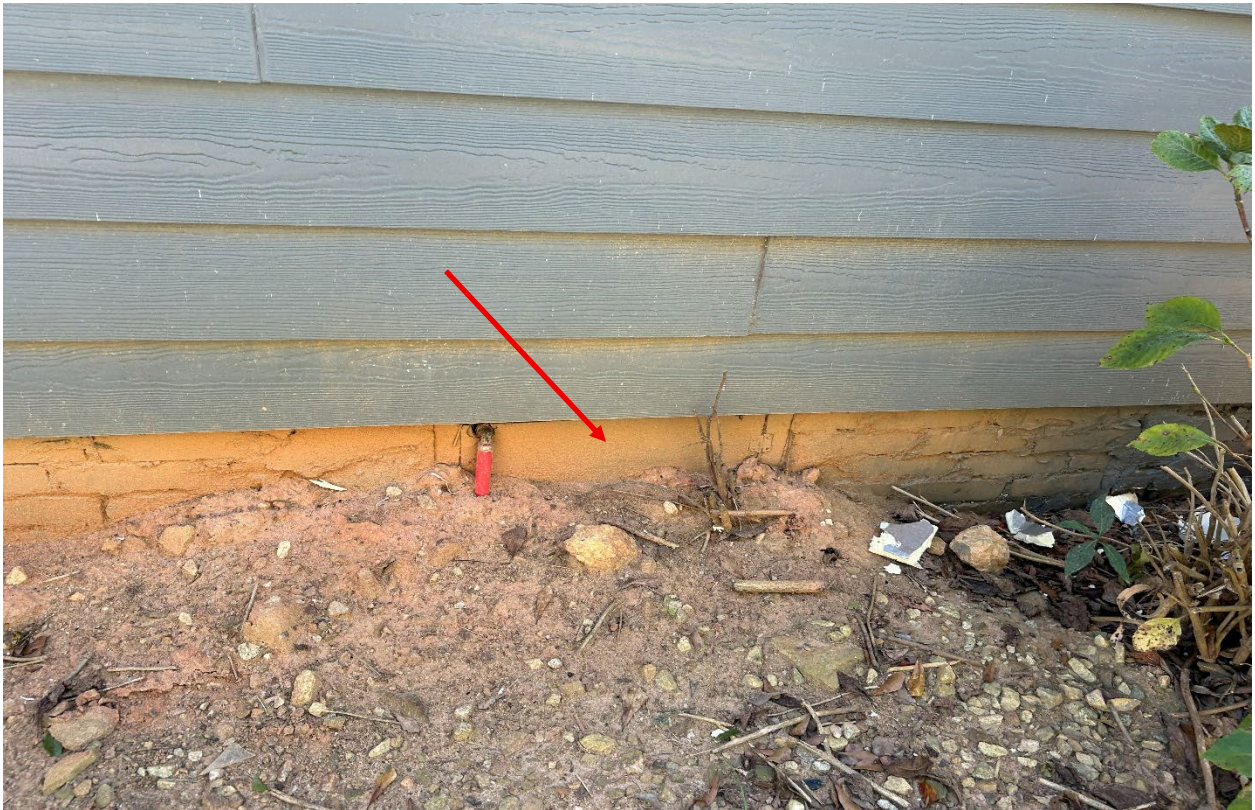
Plate 5. General photograph of the inaccessible crawlspace at the structure located at the subject property.
