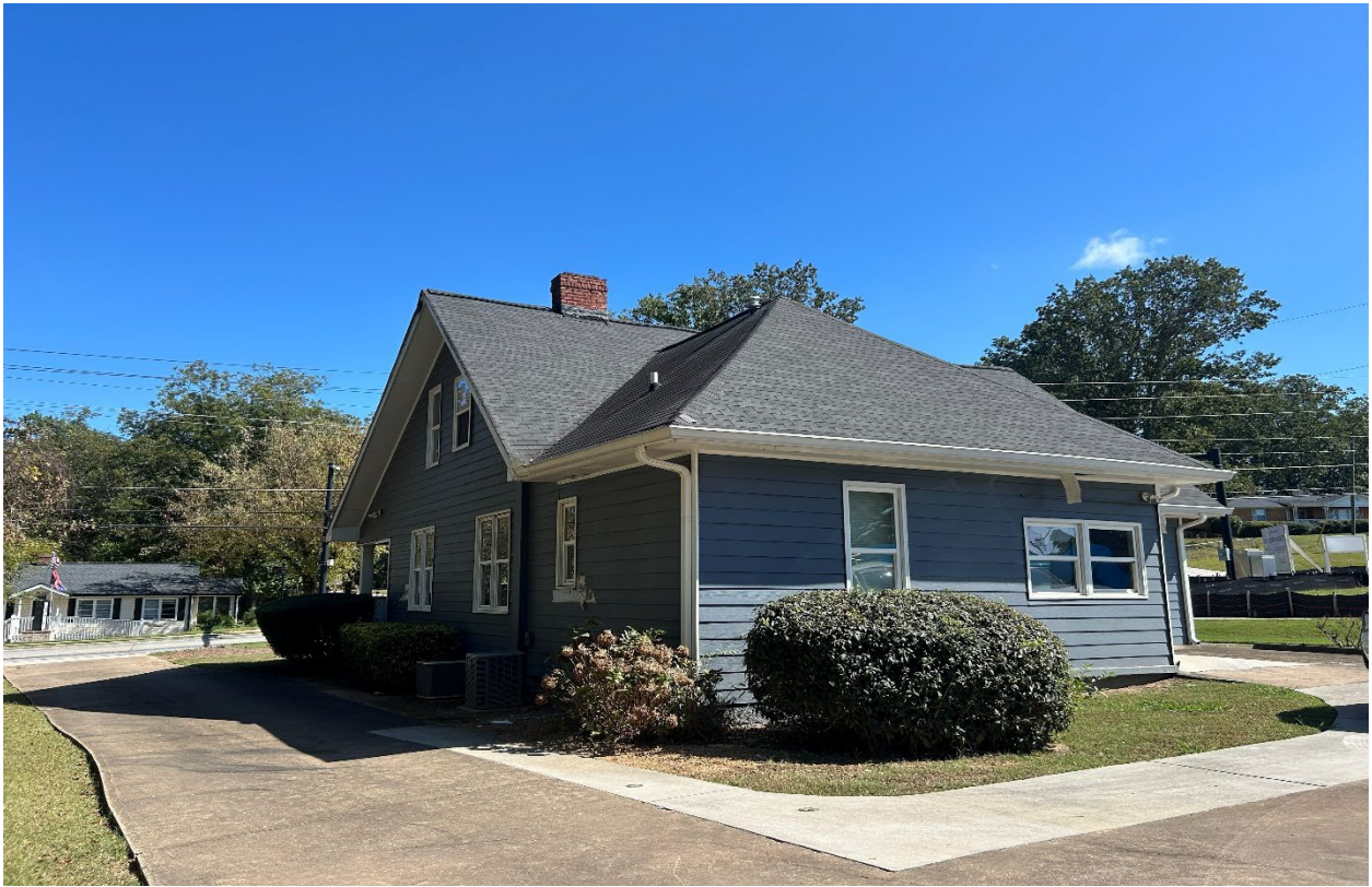
Plate 1. General photograph of the exterior of the structure located at the subject property.
