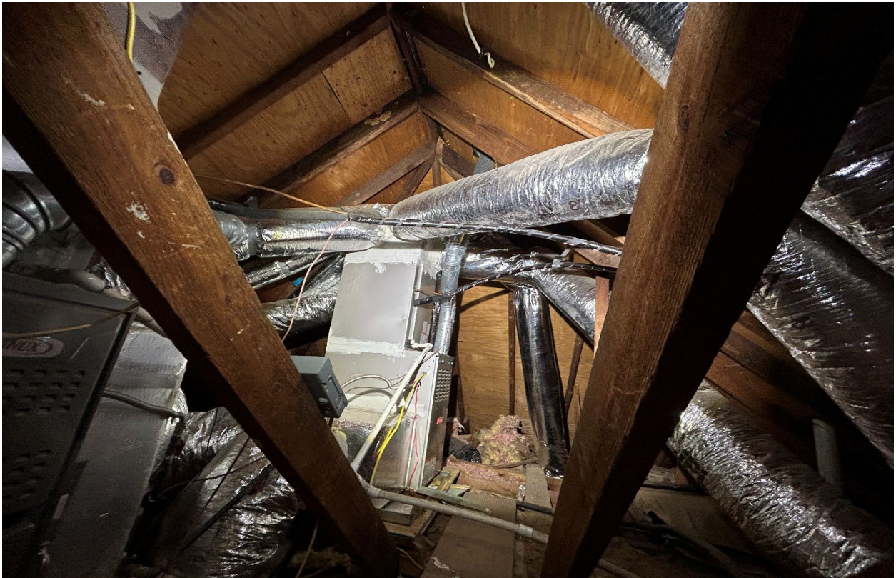
Plate 4. General photograph of the attic at the structure located at the subject property.
