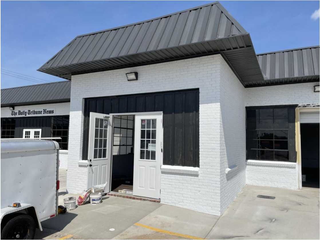
Front entrance reconfigured
