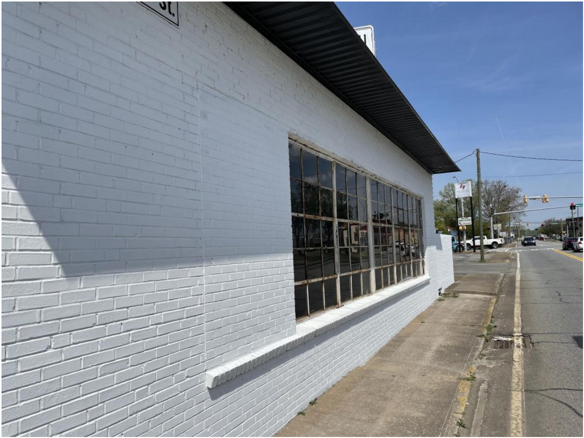
Tennessee St side. Window Opening bricked-in.
