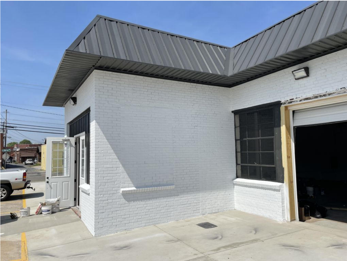
Window and standard door openings bricked-in.
