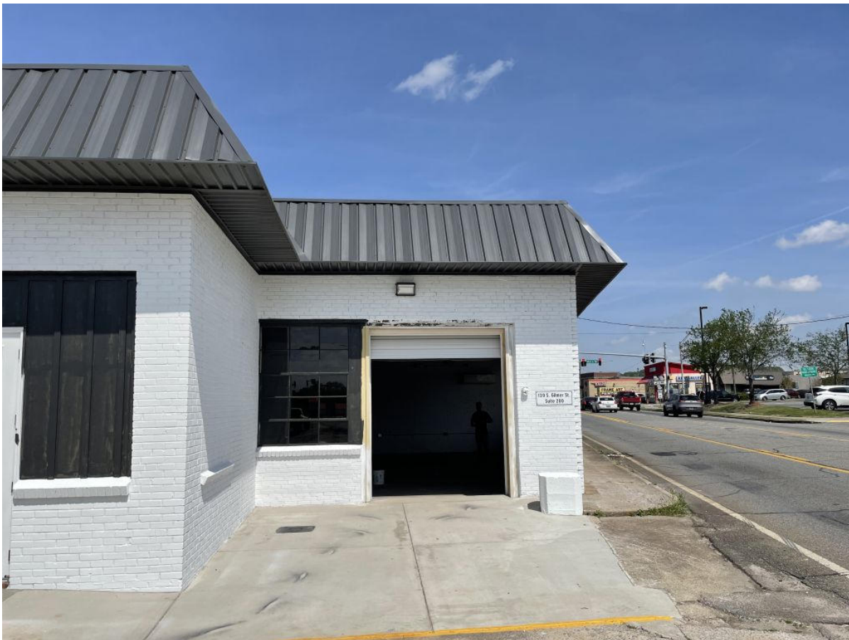
Rollup door replaced standard door with side-light windows.
