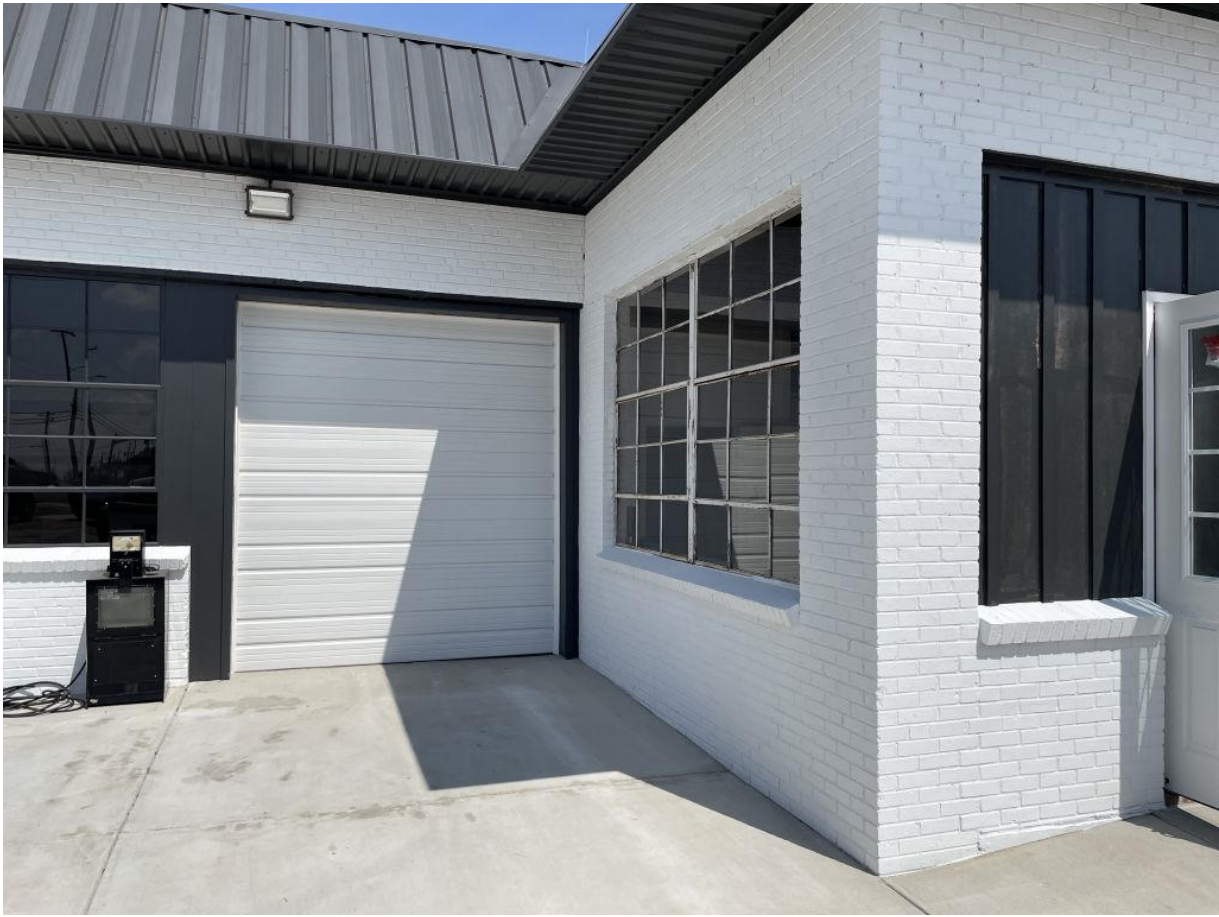
Rollup door replaced standard door with side lights
