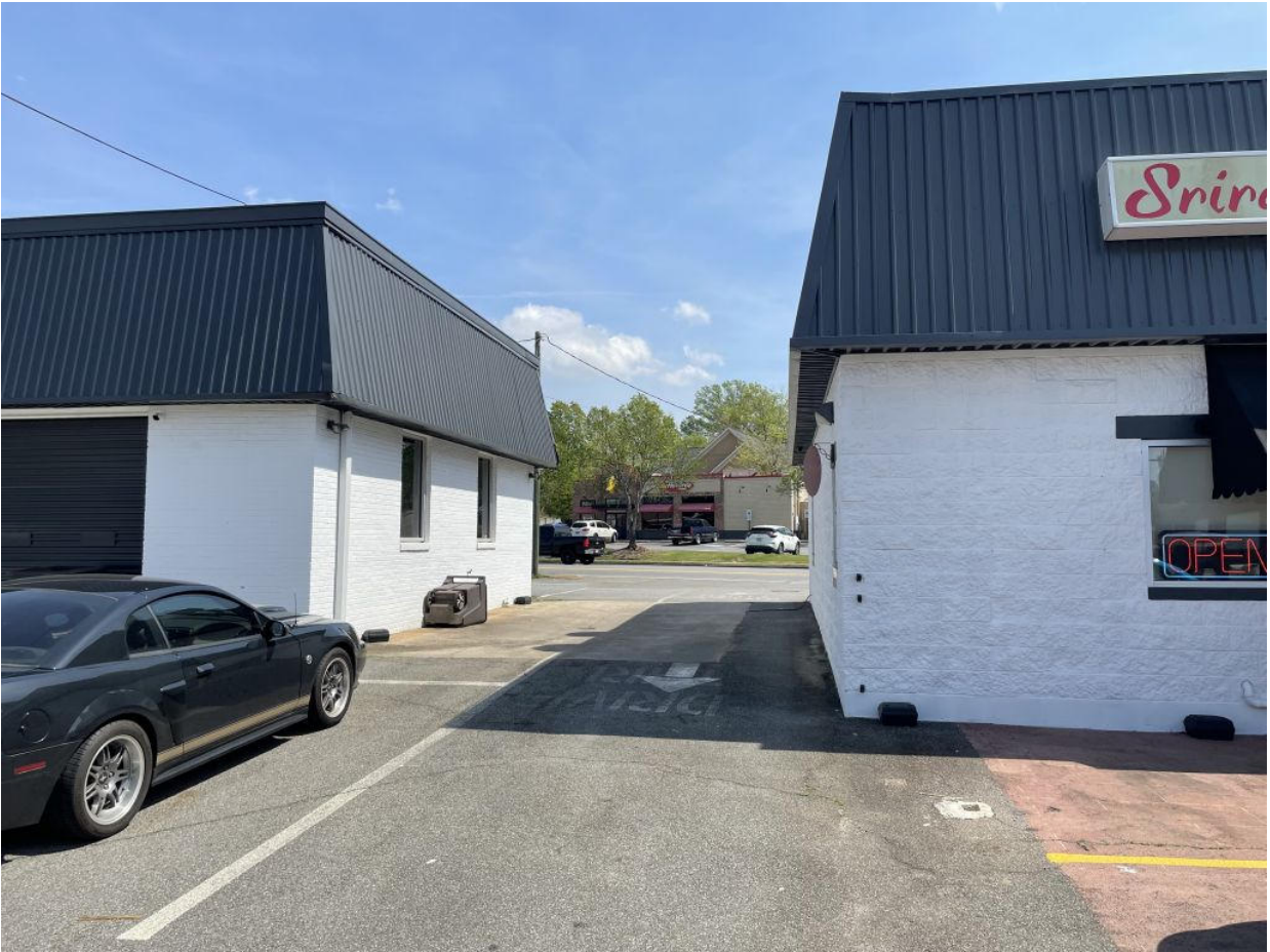
103 and 117 Building from Gilmer St.
