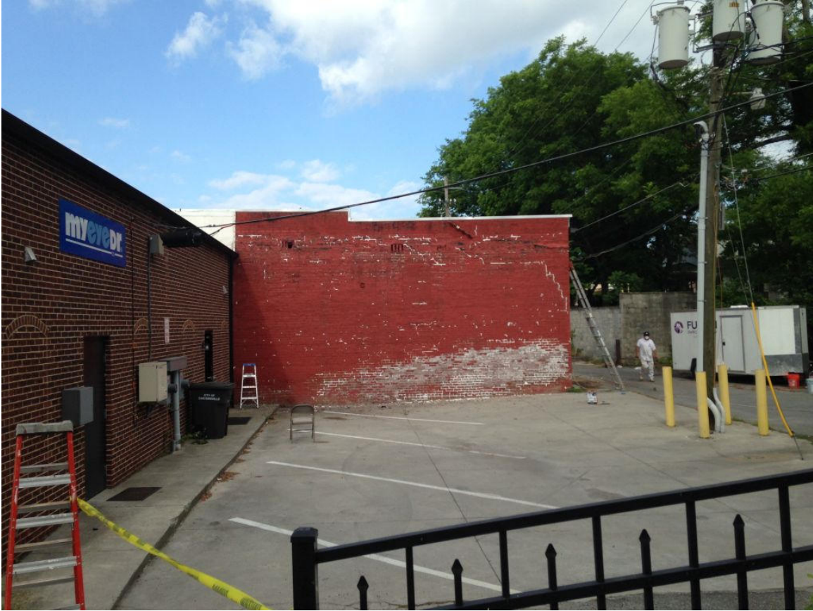
125 W. Main St. Paint removal from Brick.---Before
