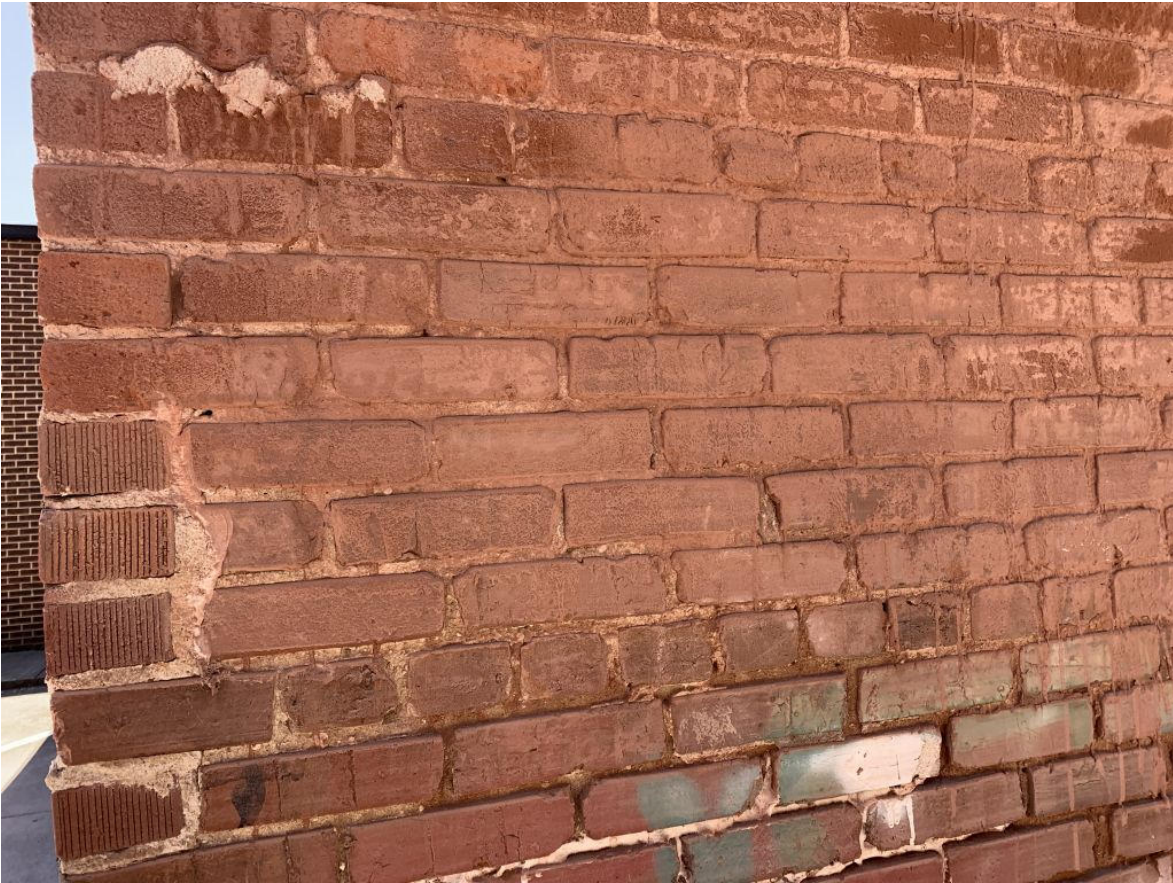
125 W. Main St. Paint removal from Brick.---After
