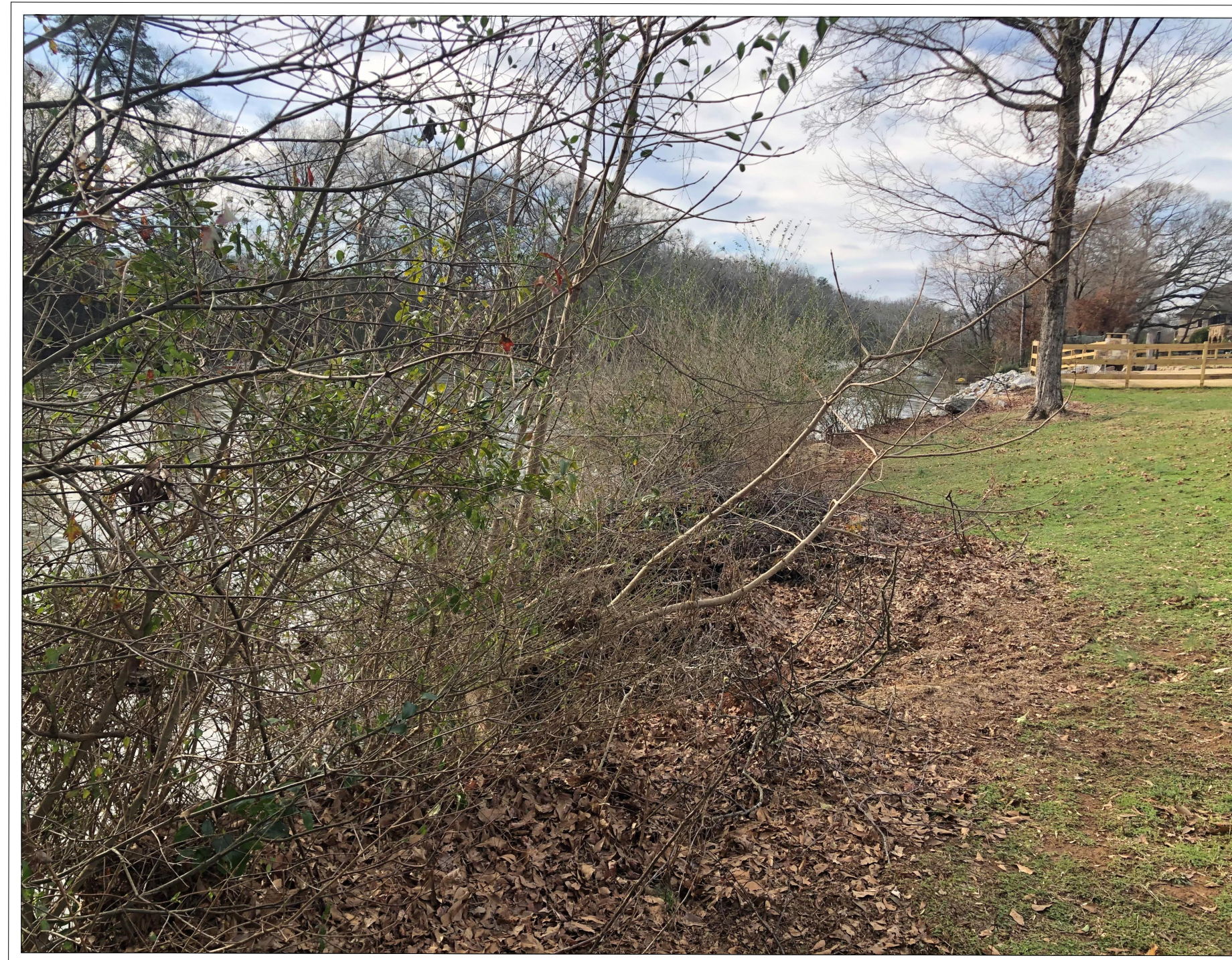
PICTURE "2" RIVER BANK ERODING
