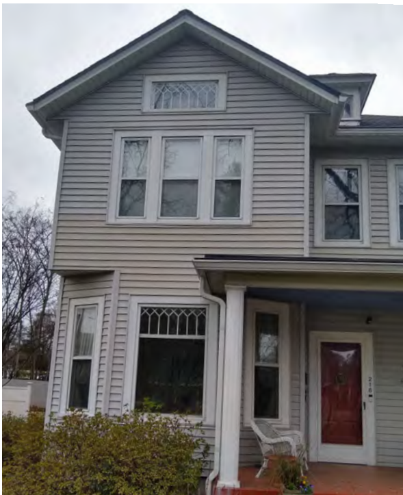
Triple window design with decorative window, Main House
