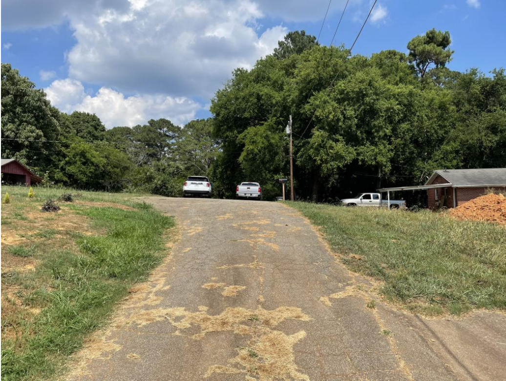
View East from midpoint of driveway. 6 Smith Rd is on the left. 7 Smith Rd is on the right ( Under renovation)
