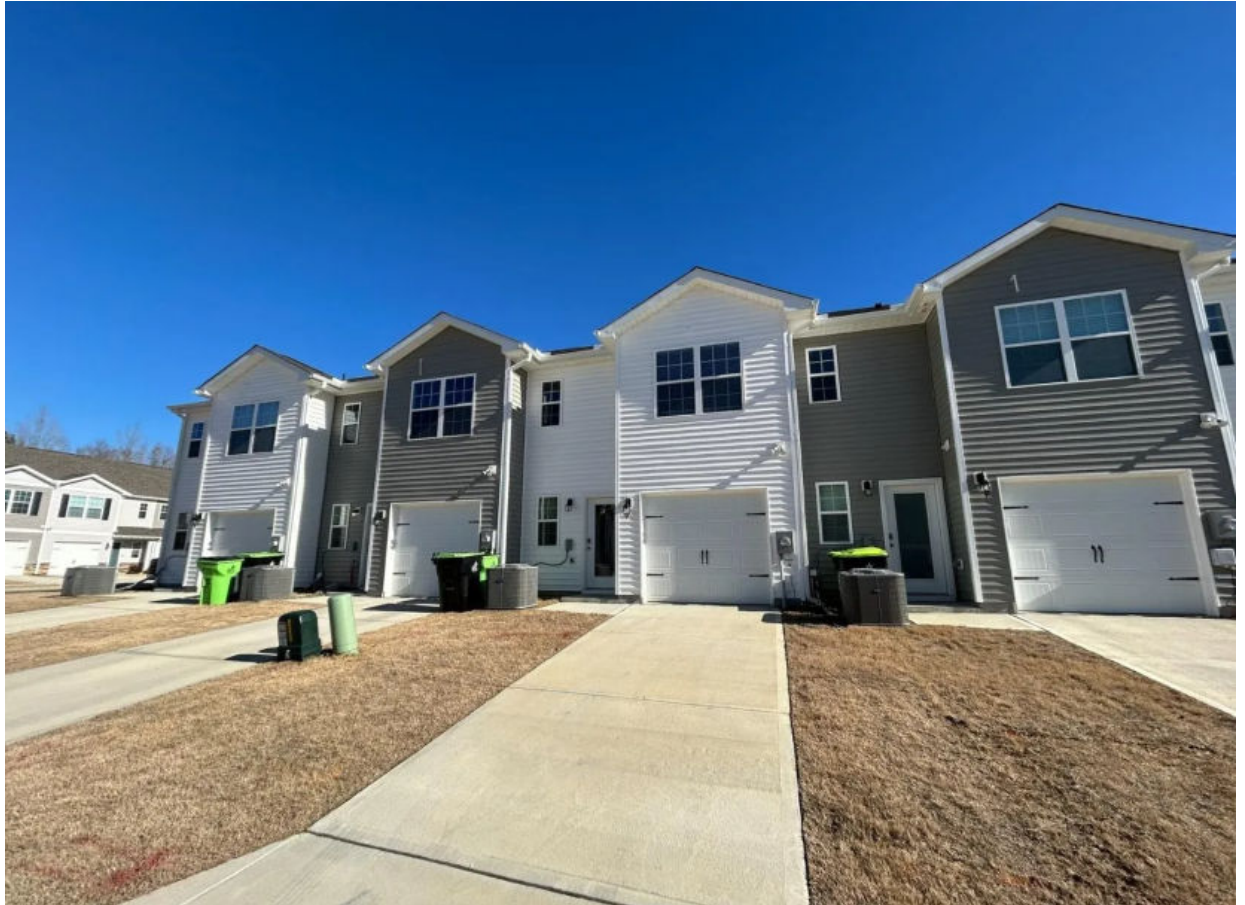
Examples from recently constructed project.
