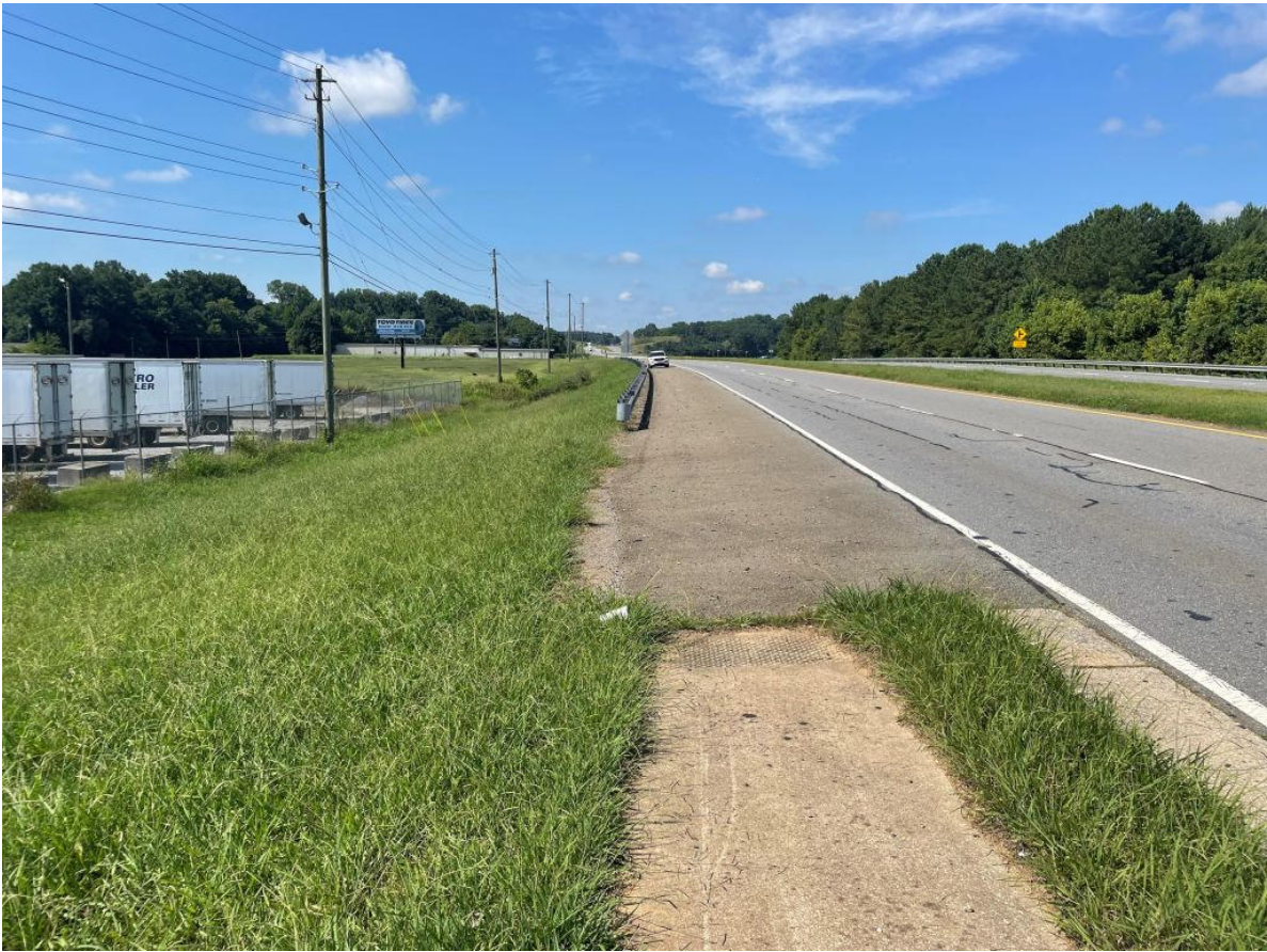
View SW from 1 River Ct. Sidewalk begins/ends. Wider shoulder.
